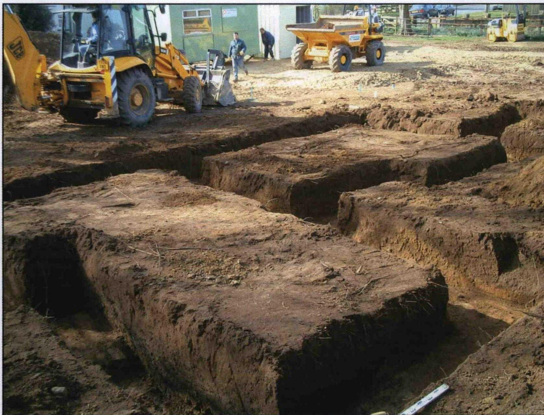
Plate 1. General view of plot 1 foundations.
