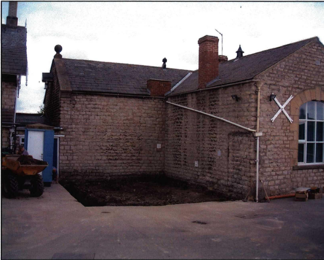
Plate 1. Location of excavation area.
