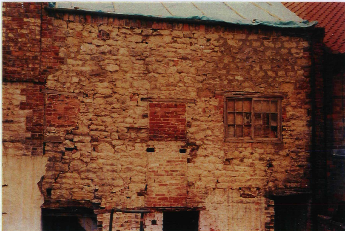
Plate 2. Detailed shot of adjacent building. Facing north.
