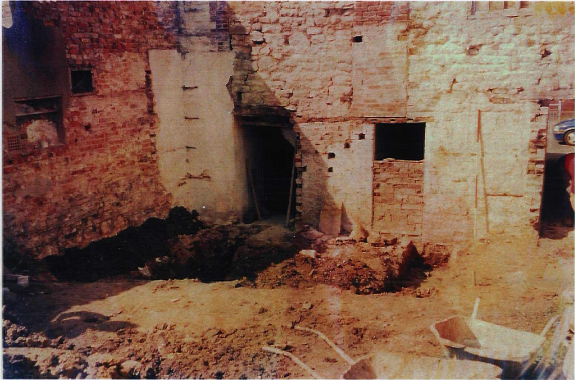
Plate 1. General shot of the site. Facing north west.
