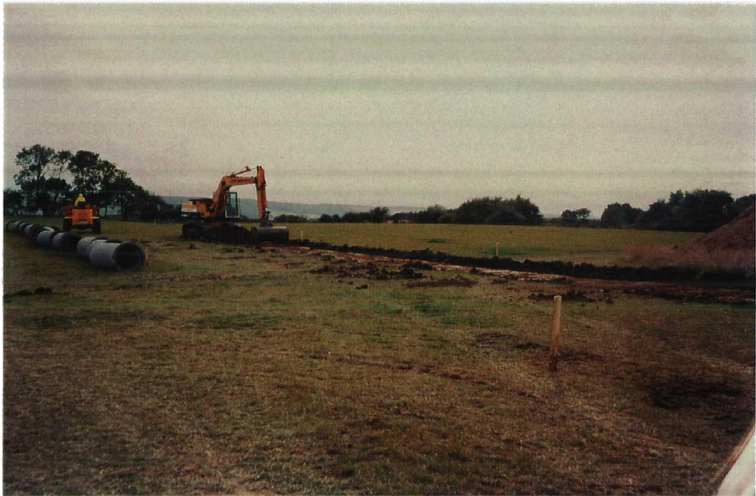
Plate 1. Topsoil stripping of the access road. Facing south west.
