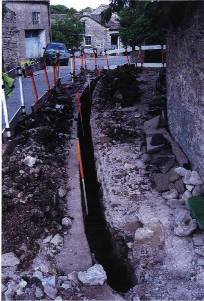
Plate 3. Excavated cable trench. Facing east.
