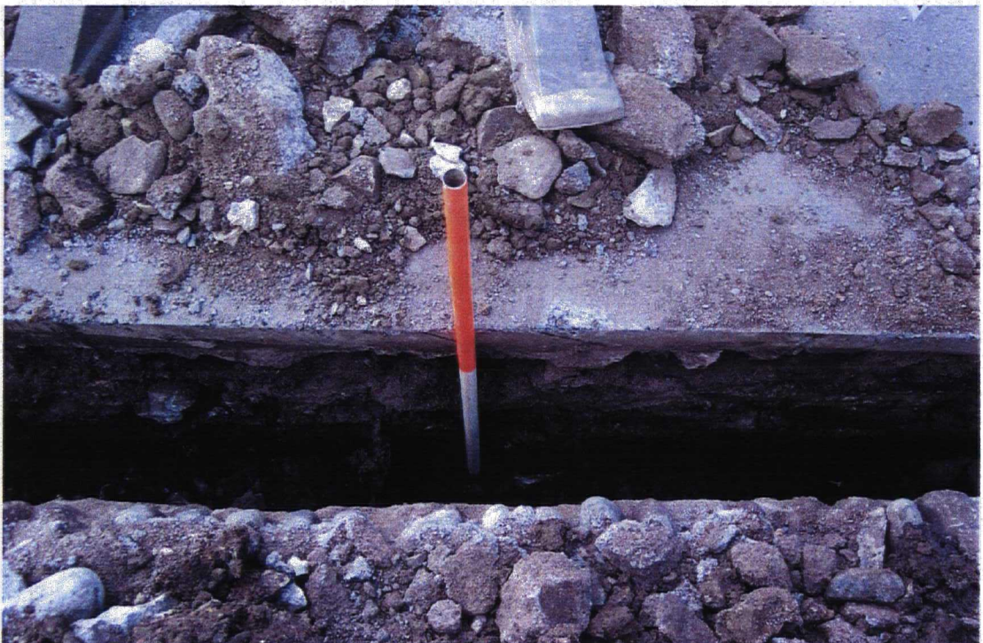
Plate 4. North facing section of excavated trench. Facing south.
