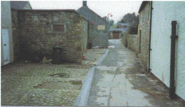
Plate 2 – Bank Yard looking west
