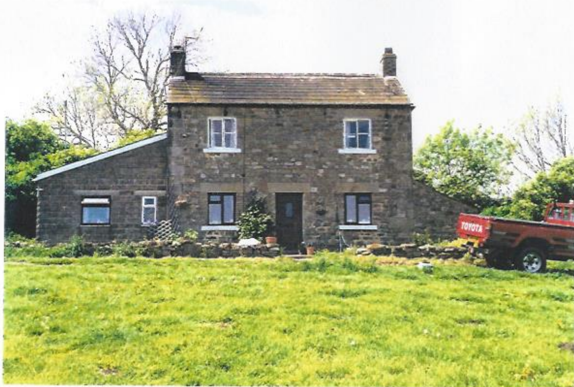
Plate 32. View of Farm house, Low Ellington, facing west.
