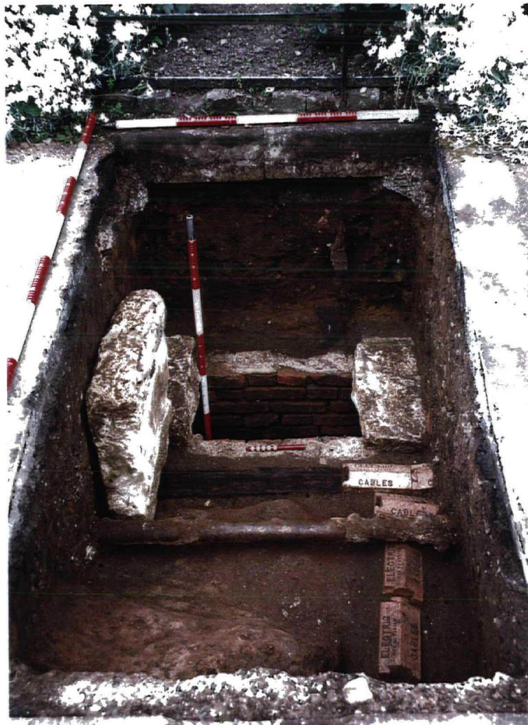
Trial Trench No.5 Internal elevation of culvert
