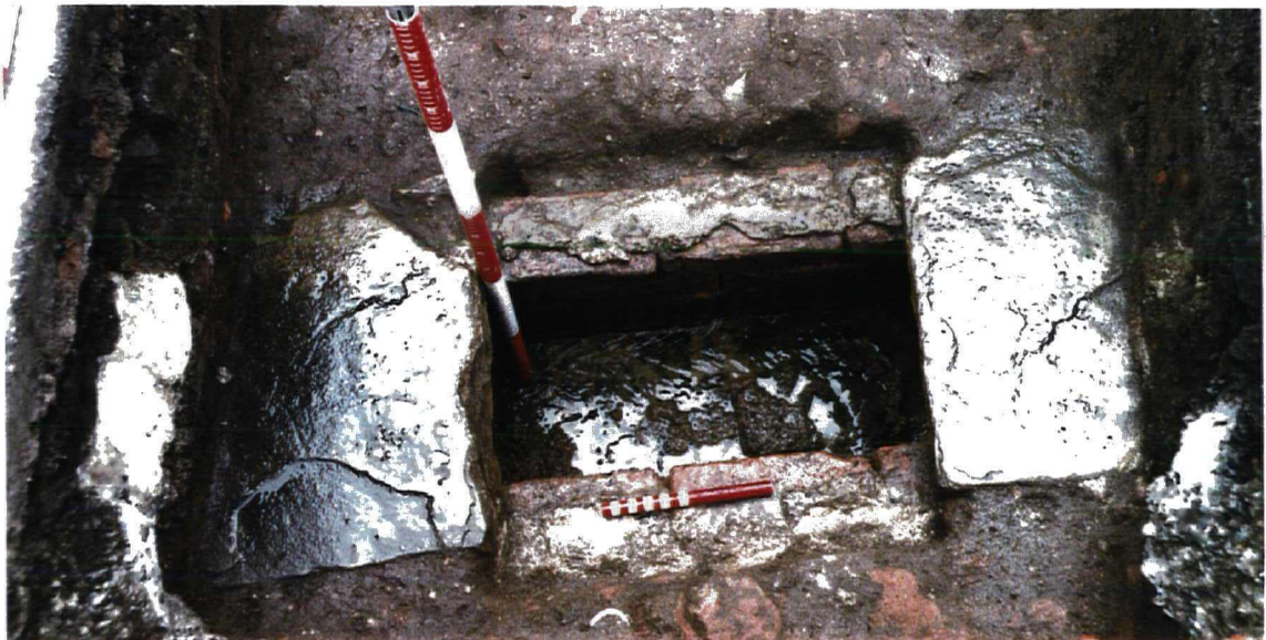
Trial Trench No.3, invert of culvert.
