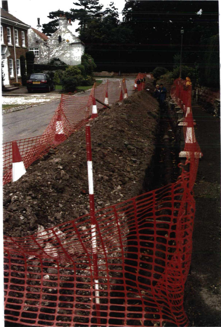
Service Trench A as excavated
