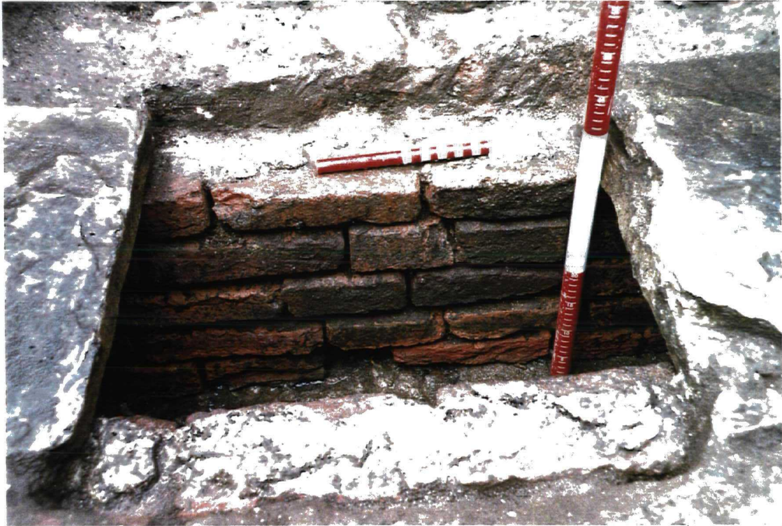
Trial Trench No.3 Detail of internal elevation of culvert
