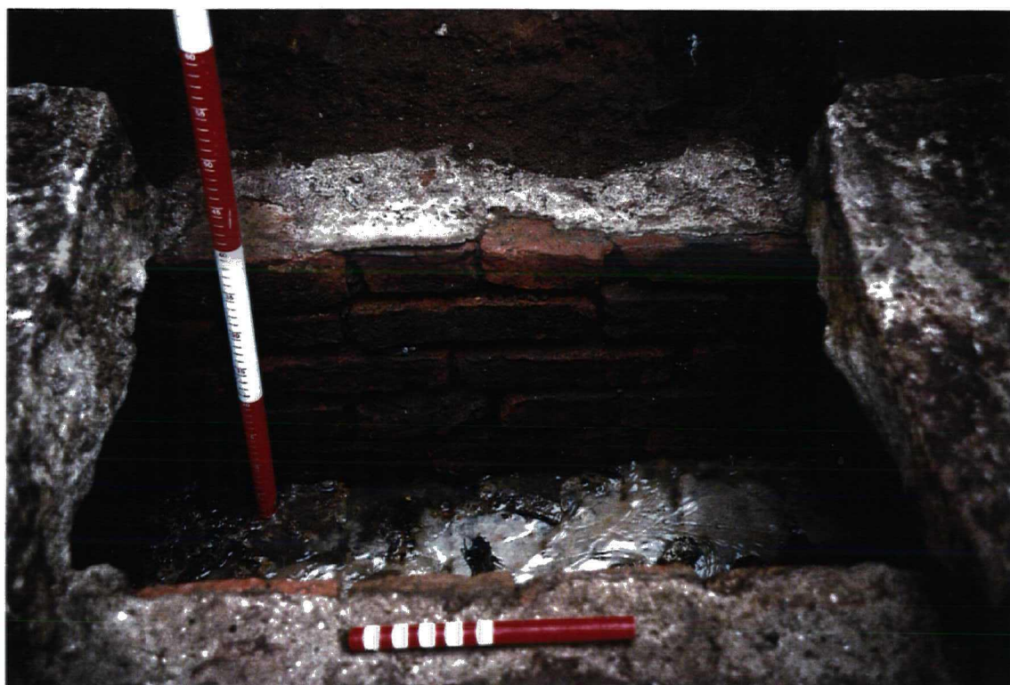
Trial Trench No.5 Detail of internal elevation of culvert
