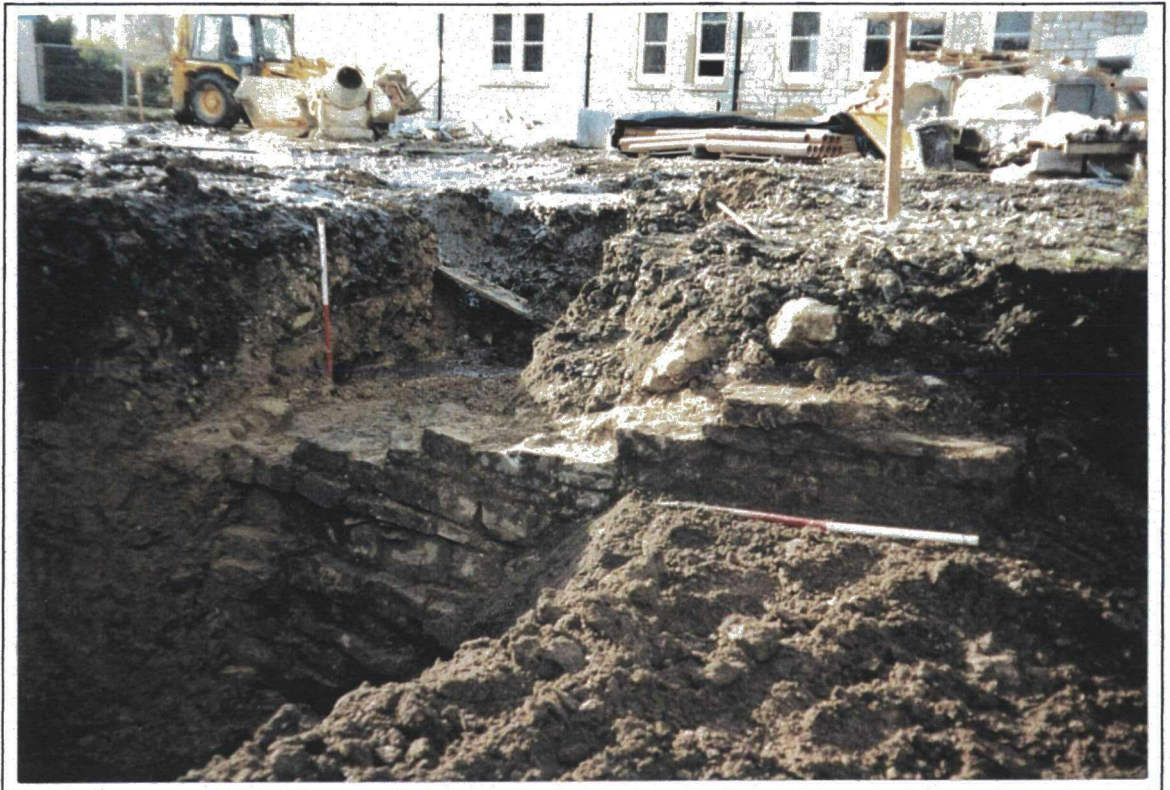
Plate 1. Wall [4] revealed in drainage trench. 2 x 1.00m scales.
