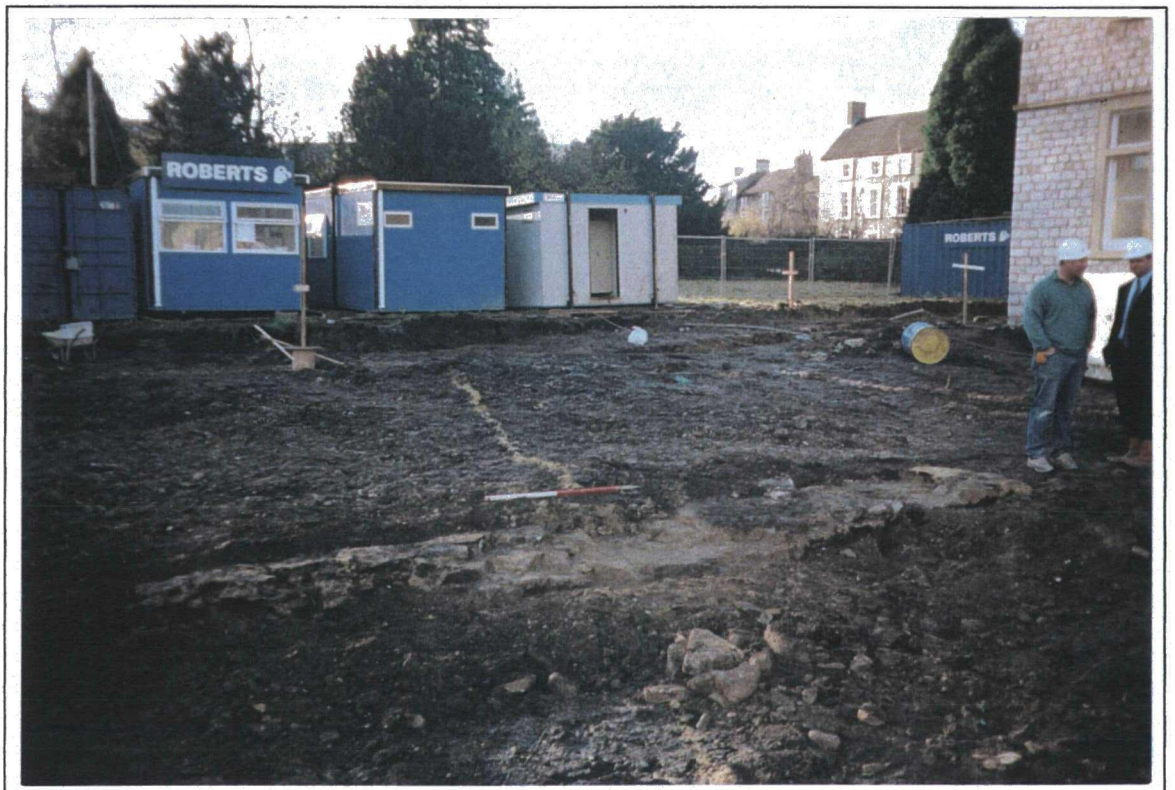
Plate 2. Wall [52] prior to excavation of drainage trench.
