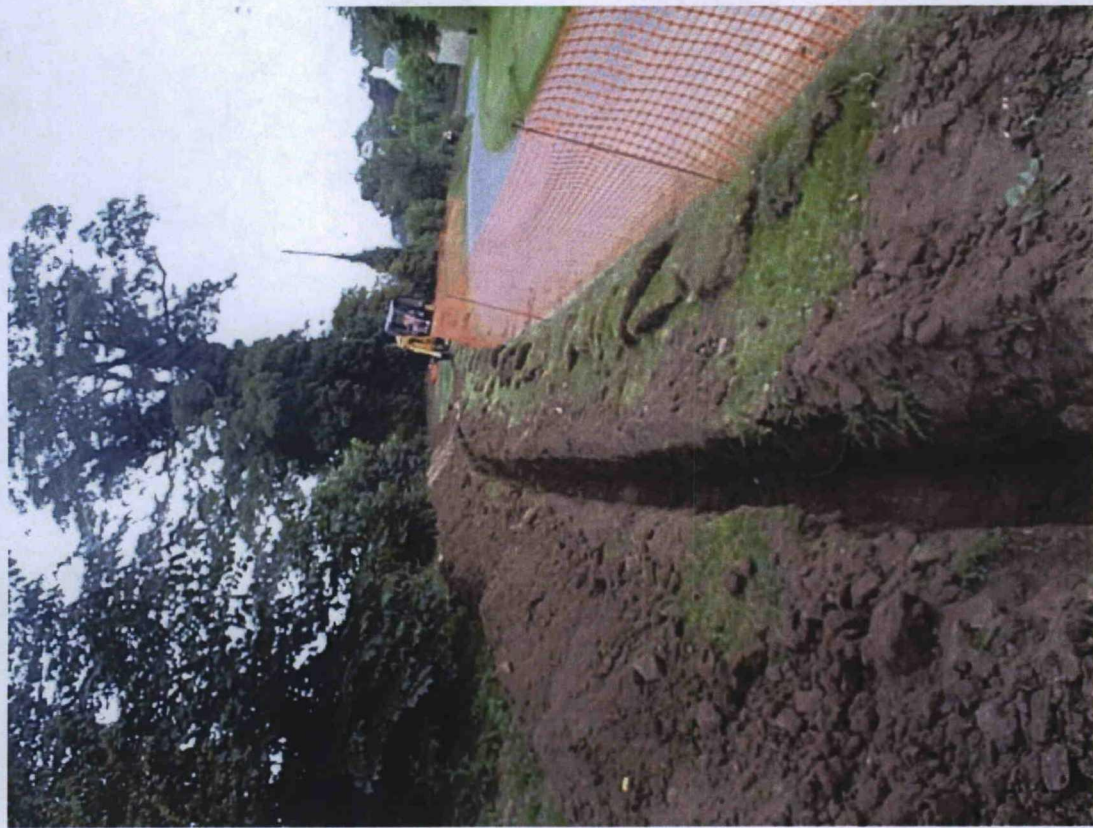
Plate 7. Burrill cable trench to east of village centre, facing East
