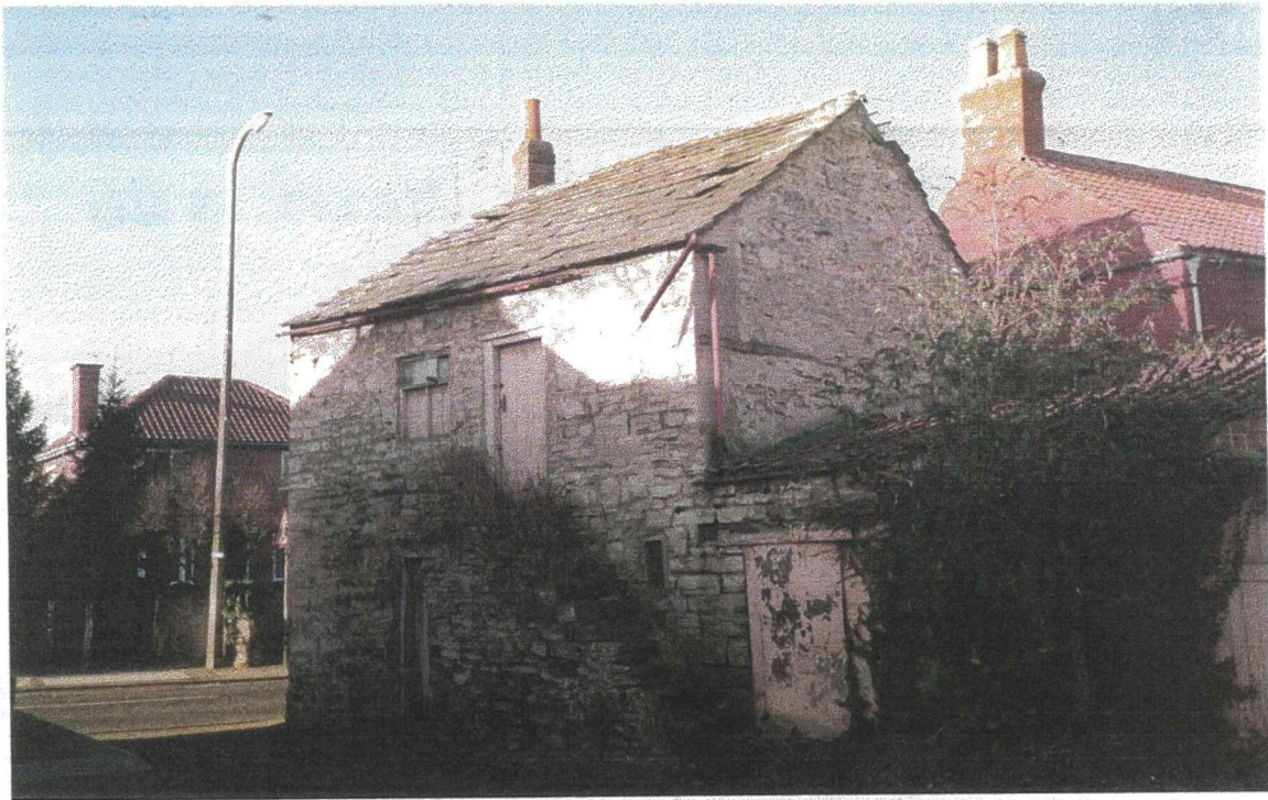
Plate 5. Farm buildings maintaining its plot on Low street. Facing north-west.
