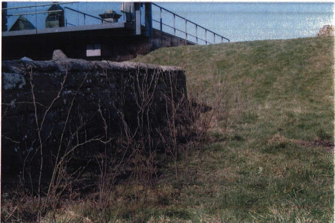
Plate 4. Completed Hedge. Facing West
