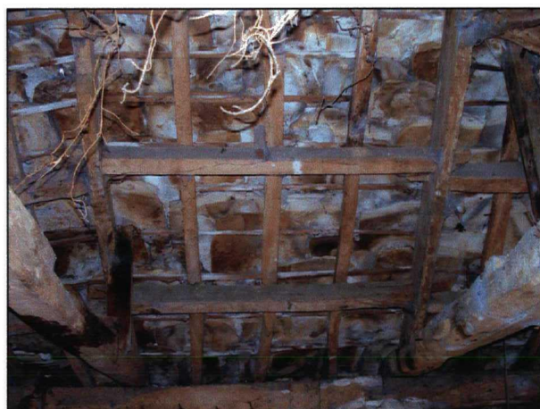
Plate 23. Roof; detail of butt purlin construction, looking west.
