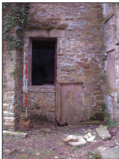
Plate 4. Early entrance to mill cut by later door, looking west. Scale of 1m.
