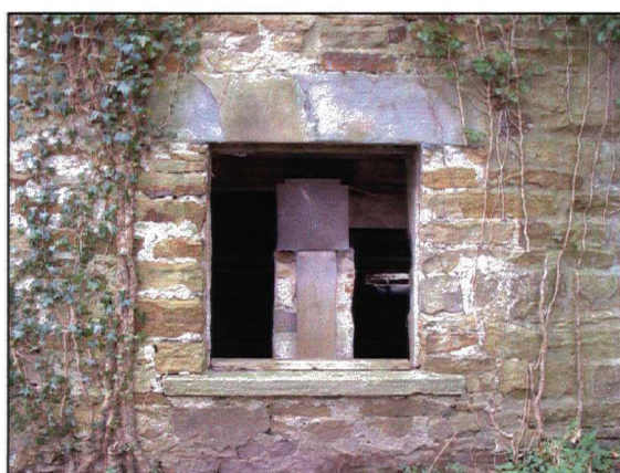
Plate 6. Window with later inserted floor beam, looking west.
