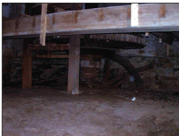
Plate 18. Mill gearing in basement; the pit wheel, looking southeast.
