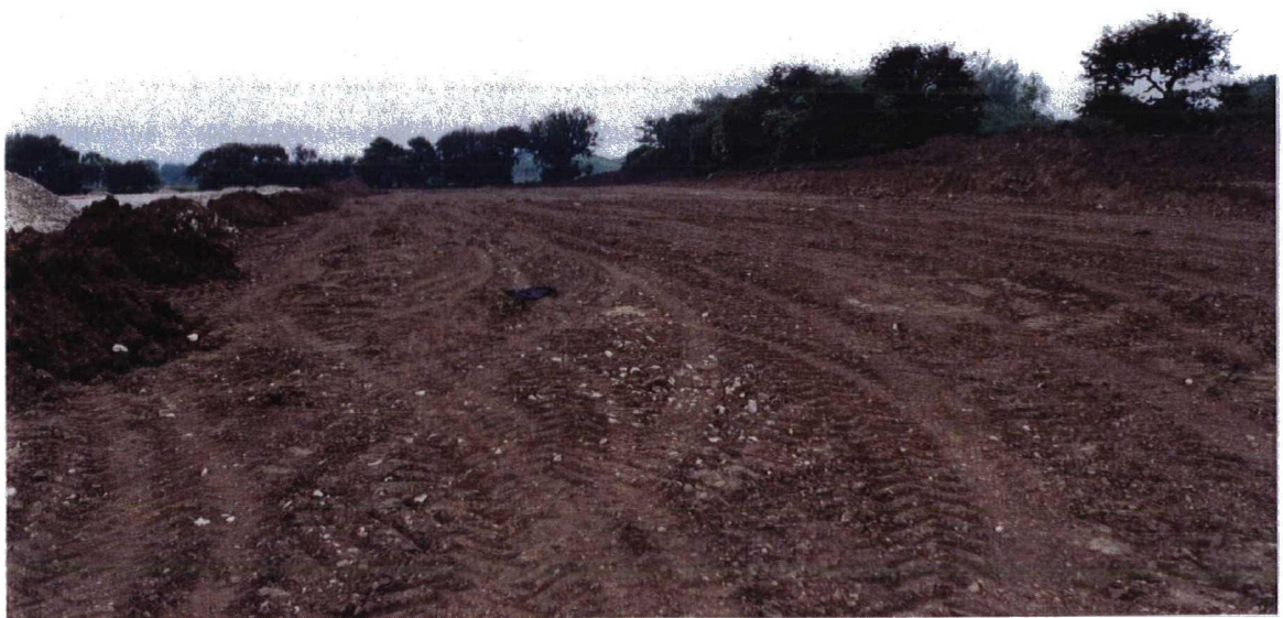
Plate 2. Site F. Area of new car park. Facing south.
