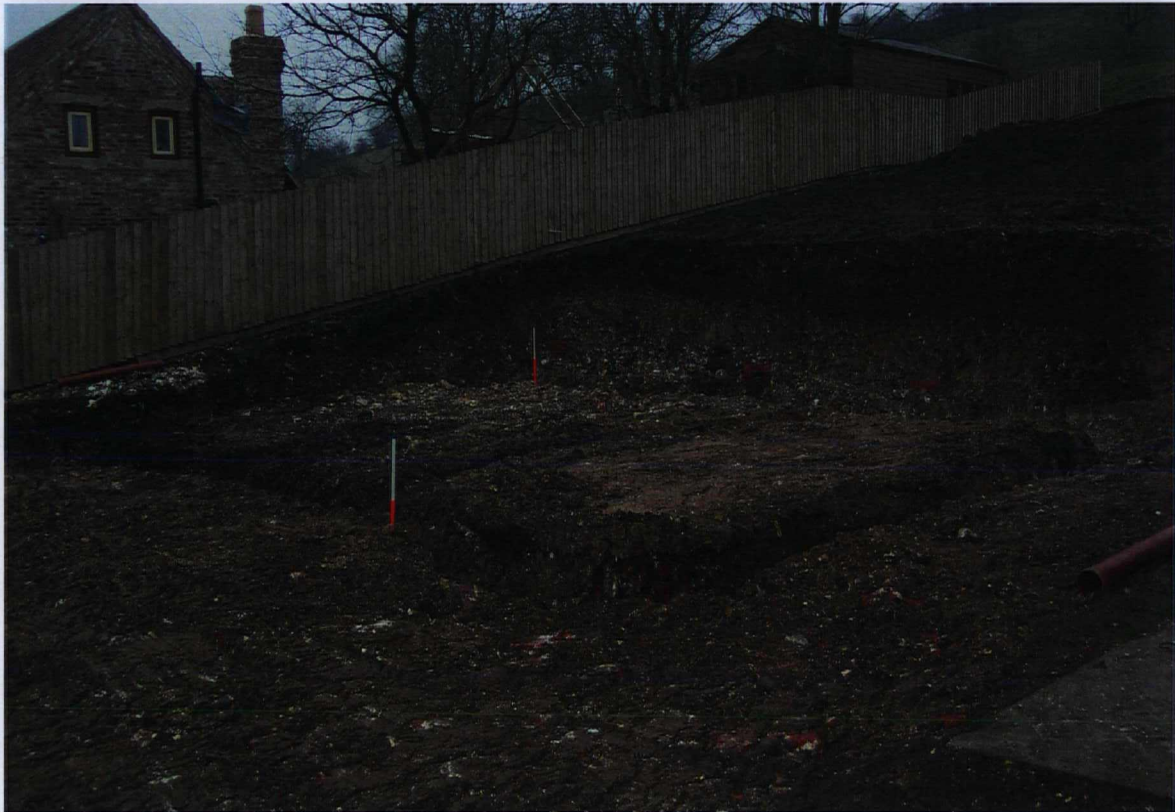
Plate 10. View of excavated footings. Facing south-east.
