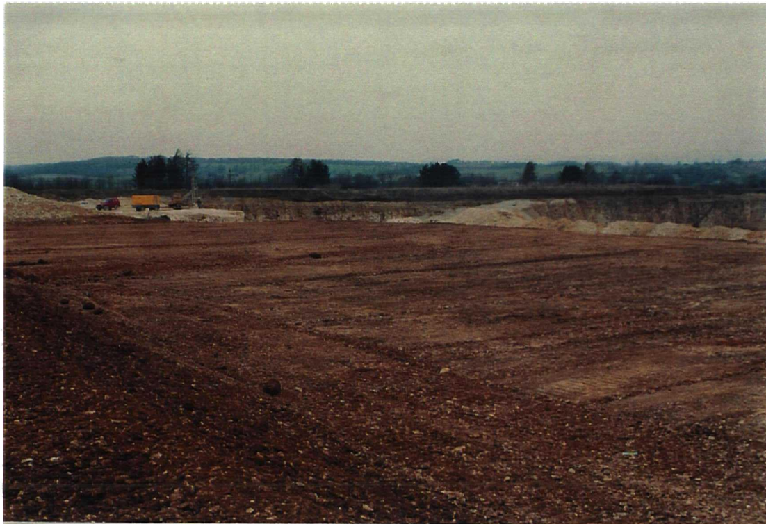
Plate 1: View of Extension Area After Topsoil Strip. Facing North-west.
