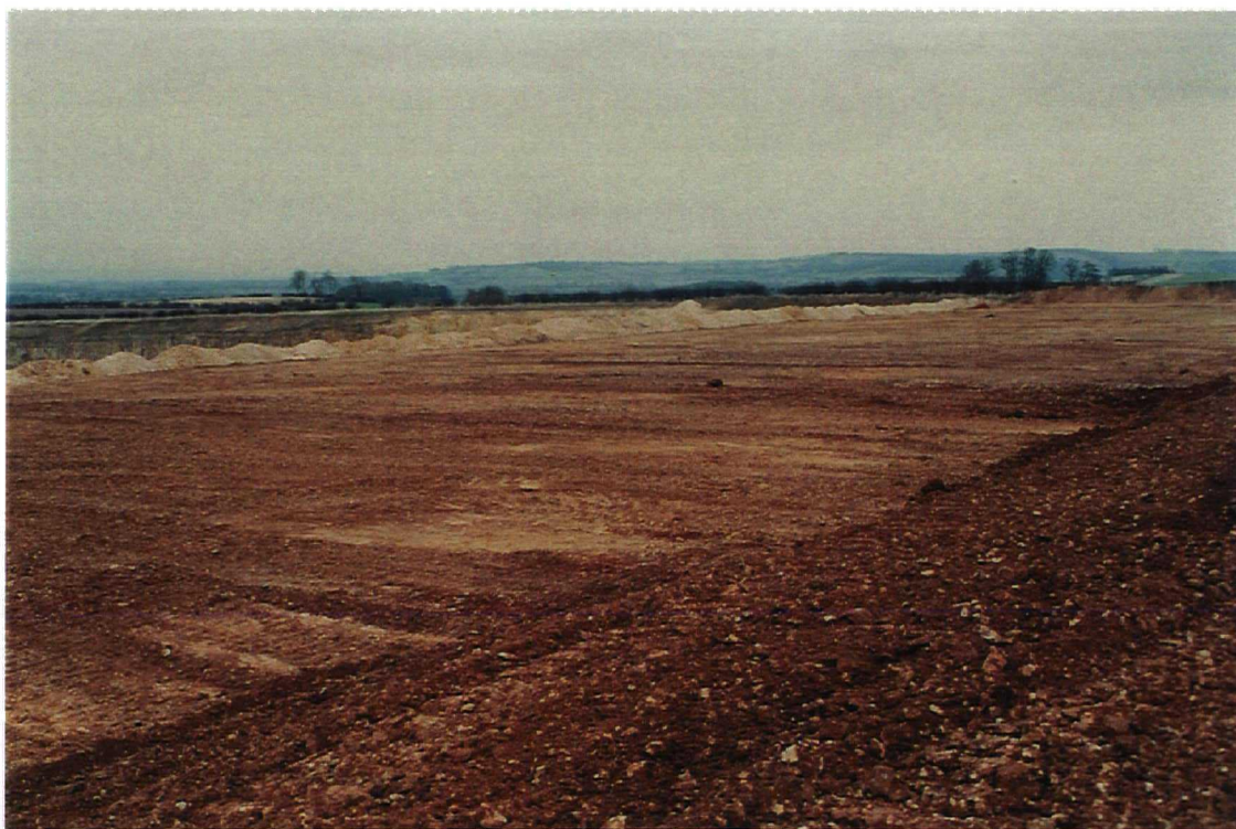
Plate 2: View of Extension Area After Topsoil Strip. Facing North-east.
