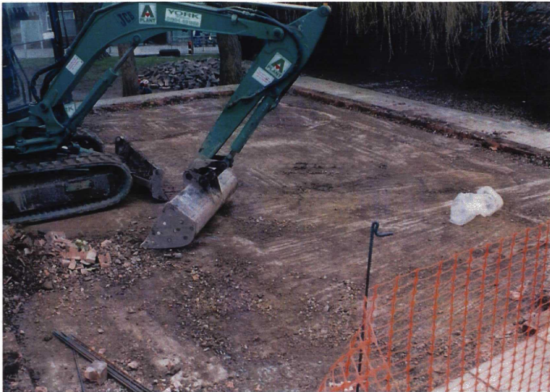
Plate 9. Working shot of Area 2 under excavation. Facing south-west.
