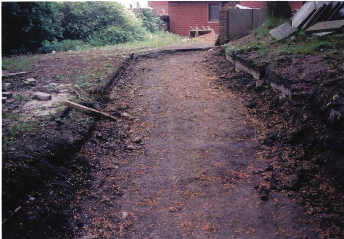
Plate 2. Area 1- North-western branch of path at finished excavation level. Facing north-west.
