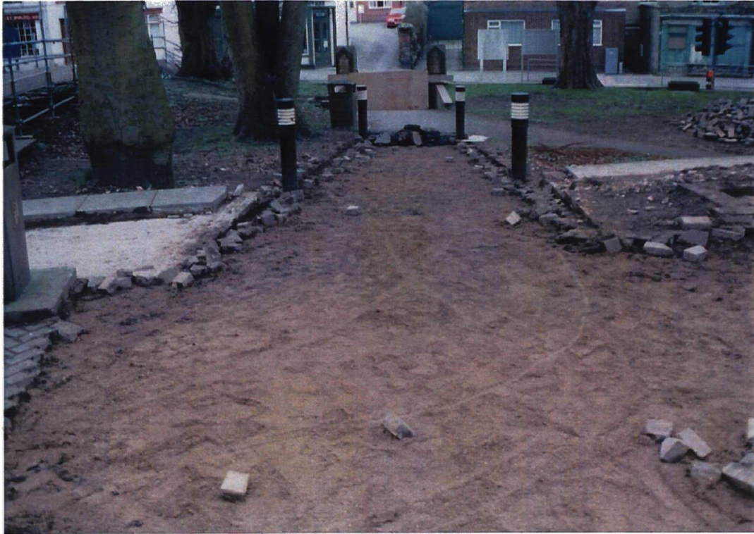
Plate 1. Area 1- Footpath after removal of surfacing. Facing south.
