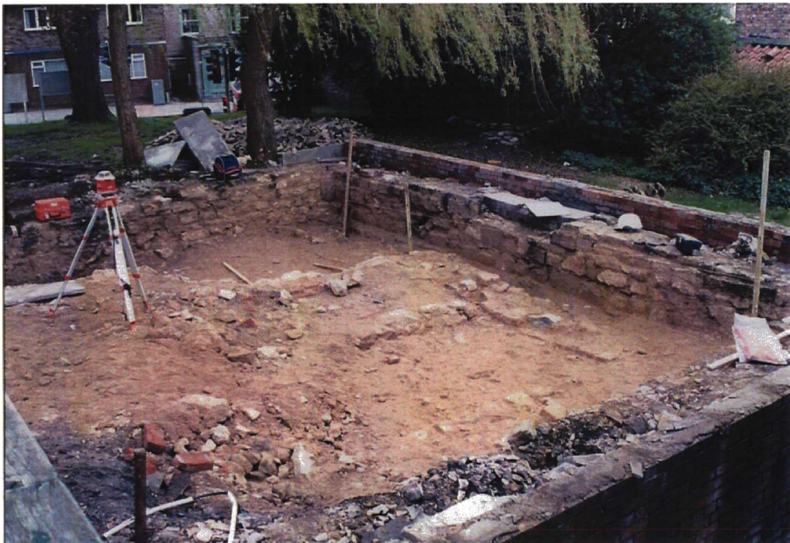
Plate 14. Area 2 showing final excavation level. Facing south-west.
