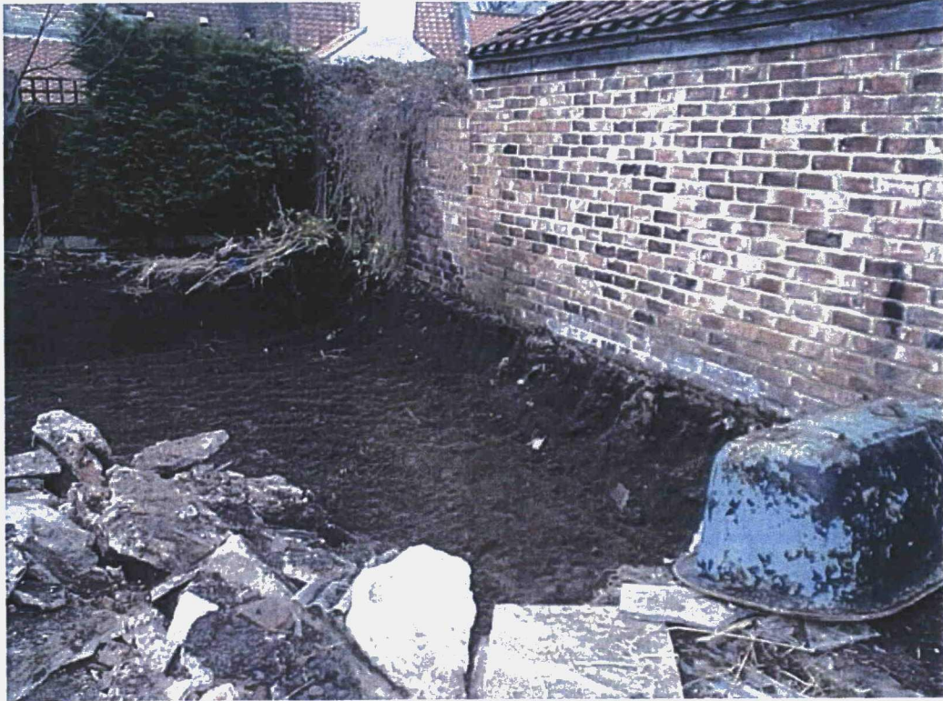
Plate 1. Excavation Work Outside Buildings, Facing North West
