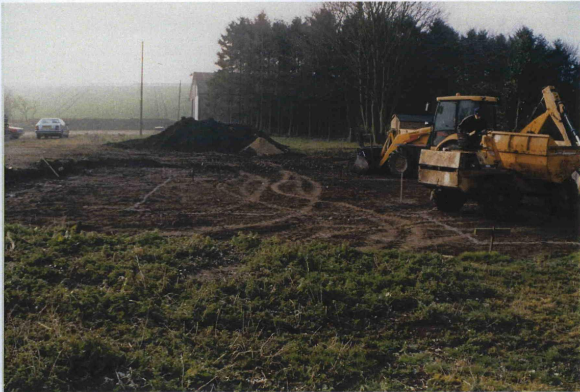
Plate 1. View of Site During Stripping. Facing South
