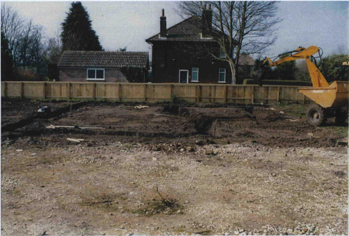
Plate 3. View of Excavated Footings. Facing West
