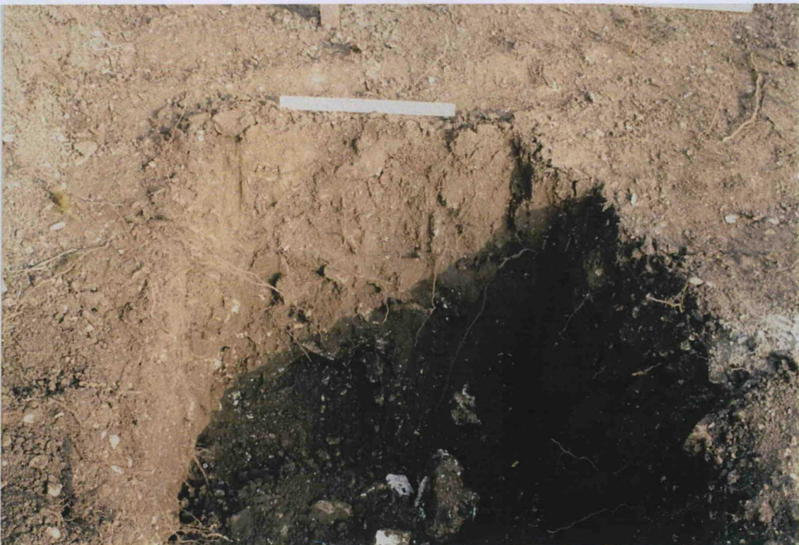
Plate 4. Excavated Footing. Facing South
