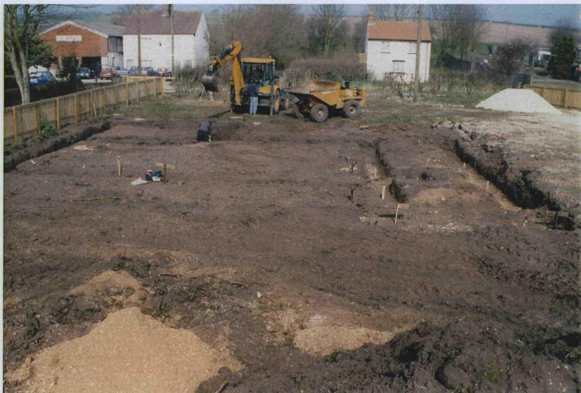
Plate 2. View of Excavated Footings. Facing North North West
