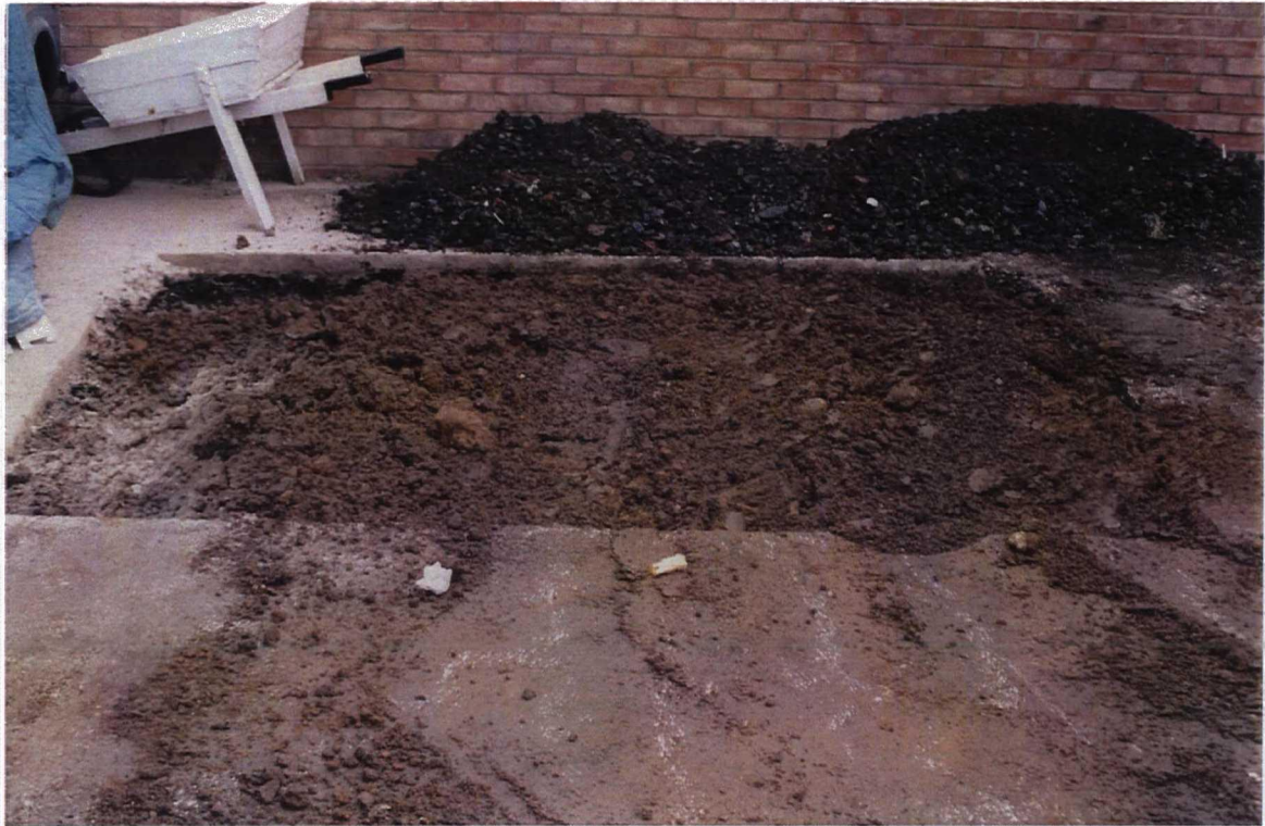
Plate 1. Excavation Trench During Excavation, Facing East
