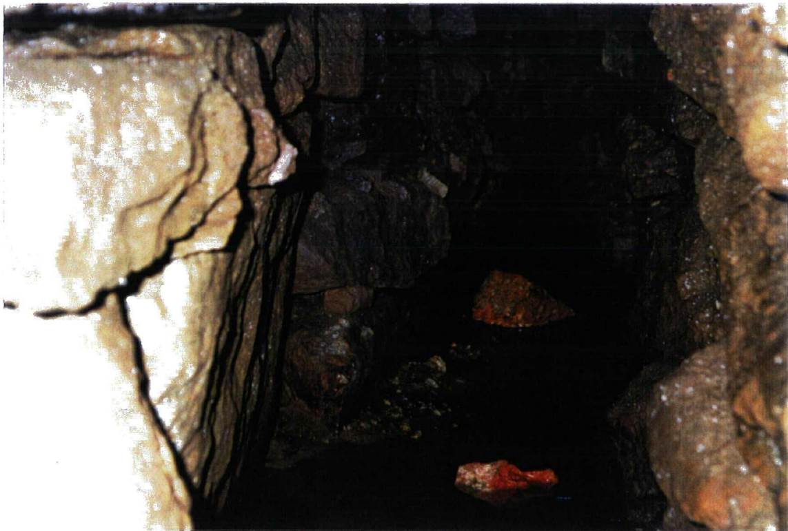
Plate 6 View of base of inner culvert 1006. Facing south.
