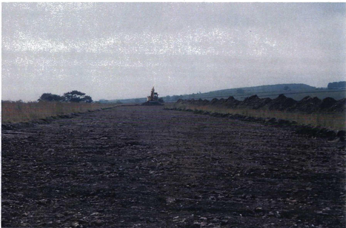
Plate 2. General view of topsoil strip. Facing East
