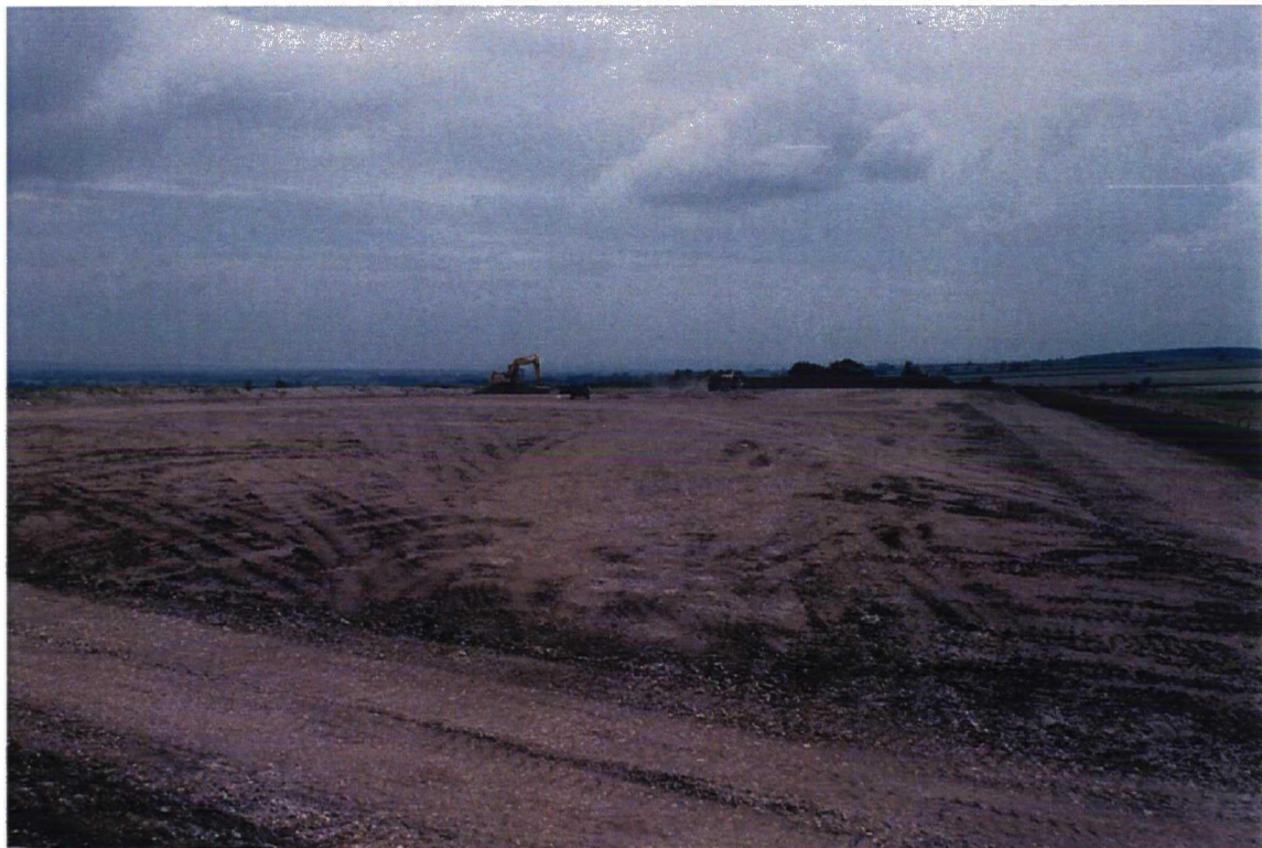
Plate 10. General view of topsoil strip. Facing North-east
