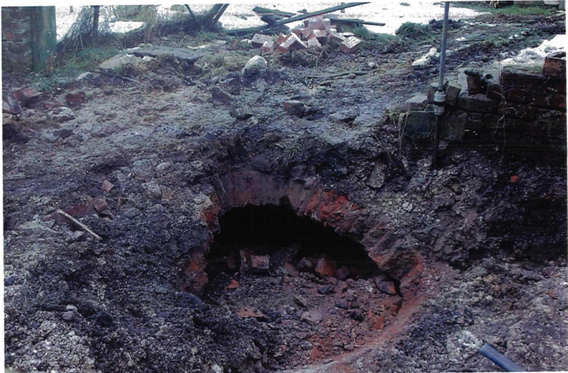
Plate 3. Domed Brick Structure, After Partial Demolition, Facing North East
