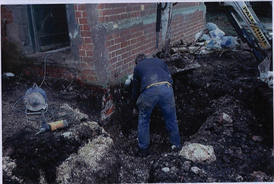
Plate 6. Foundation Trench After Removal of Wall, Facing West South West
