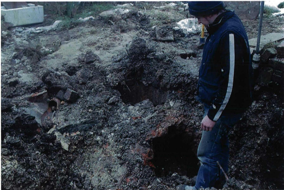
Plate 2. Domed Brick Structure, Facing North East
