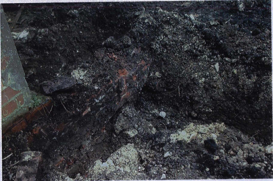
Plate 5. Wall, Facing North West
