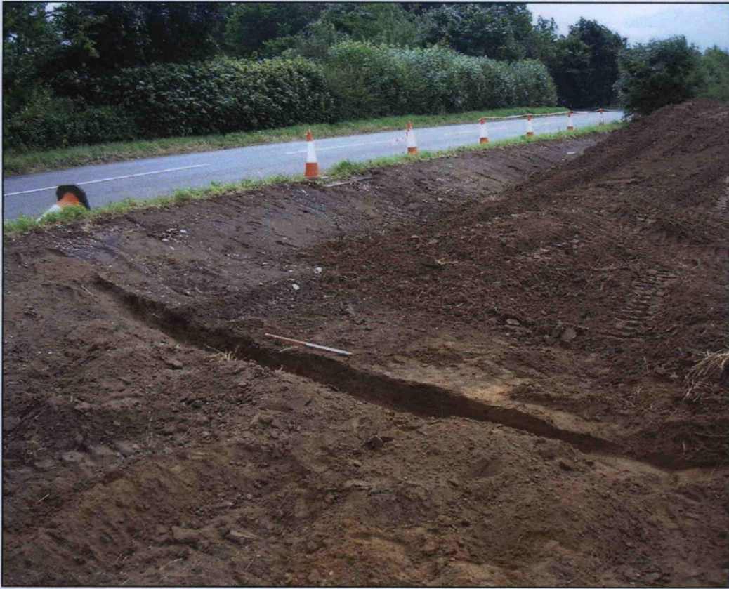
Plate 3. Section through roadside ditch [603], looking southeast. (Scale of 2m).
