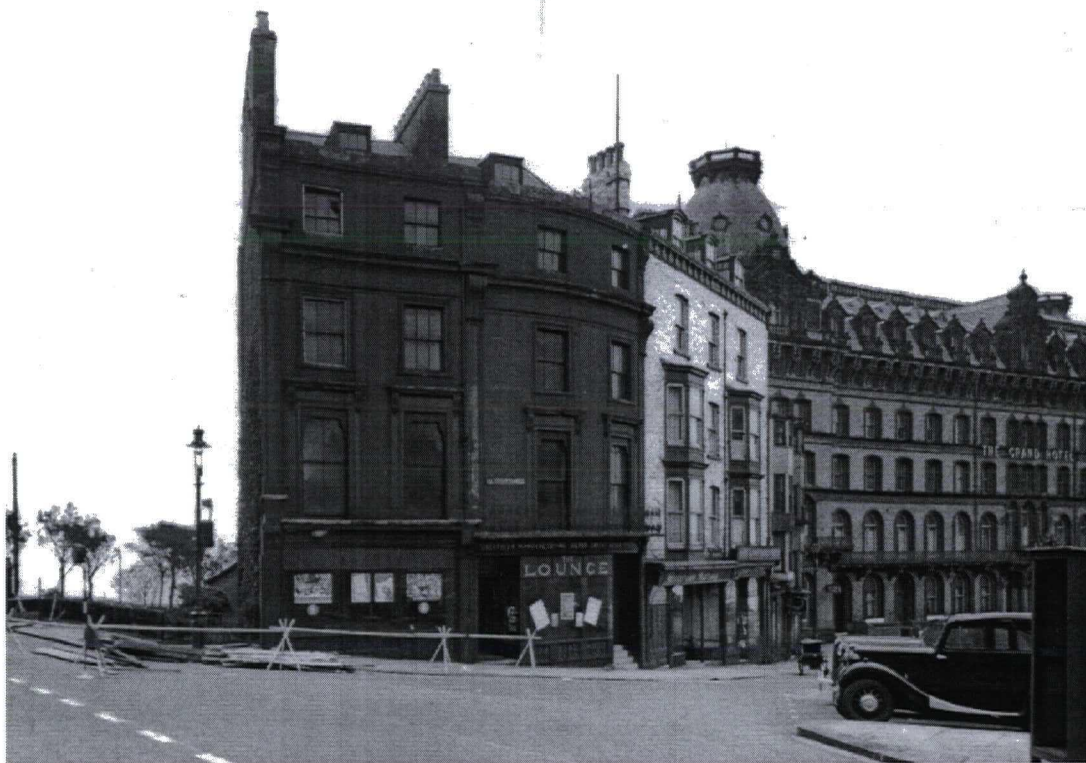
The site on 9 October 1939 as demolition of The Lounge commences
