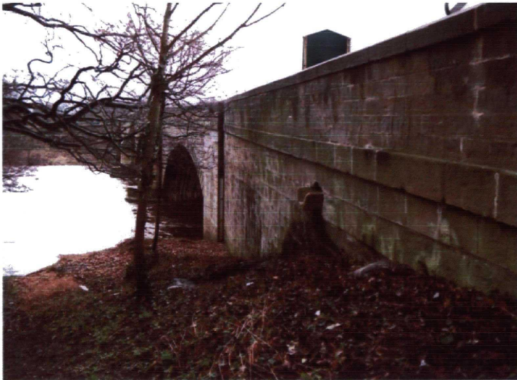
Plate 2, The east side of Tanfield Bridge, from the north bank of the River Ure, showing the drain carrying run-off water
