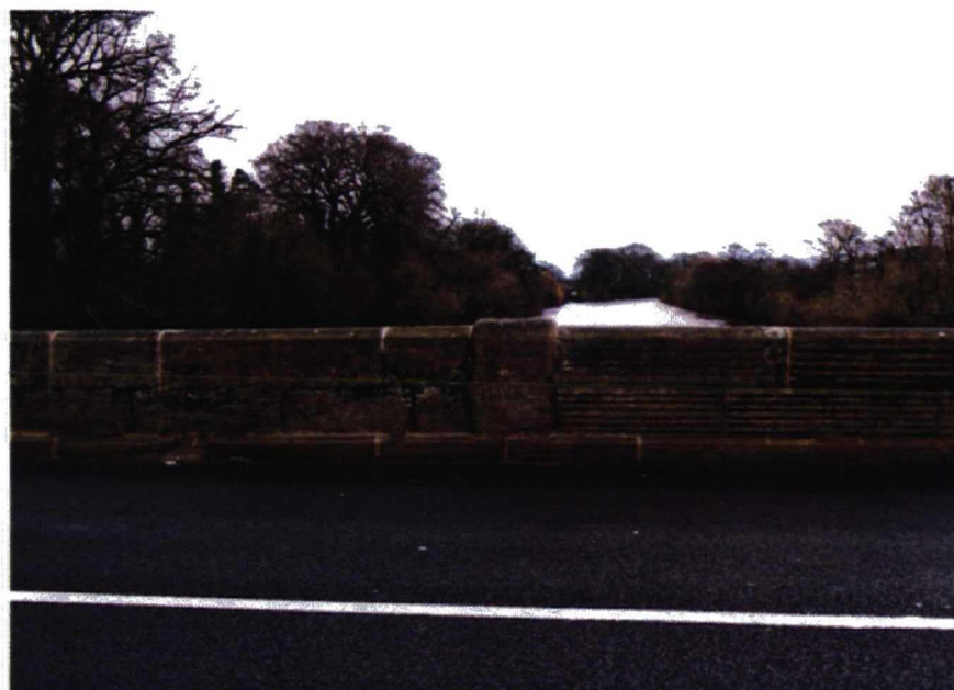
Plate 2: The inner, west side of Tanfield Bridge from showing the division between the North and West Ridings
