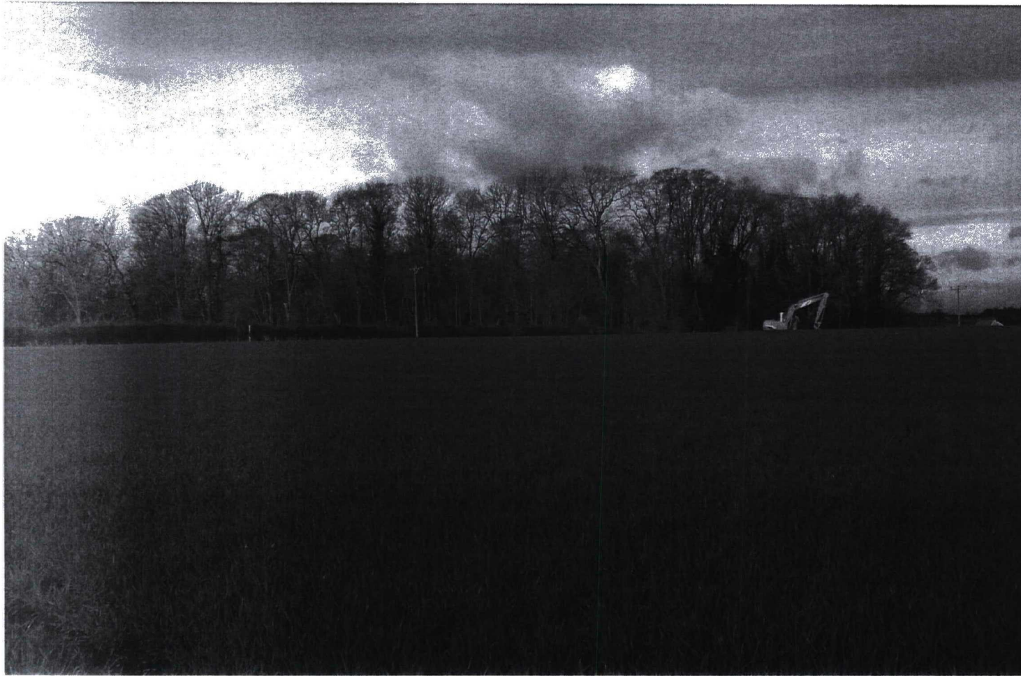
Plate 9. Alignment of Trench 1 pipe trench, prior to excavation. Facing north-west.
