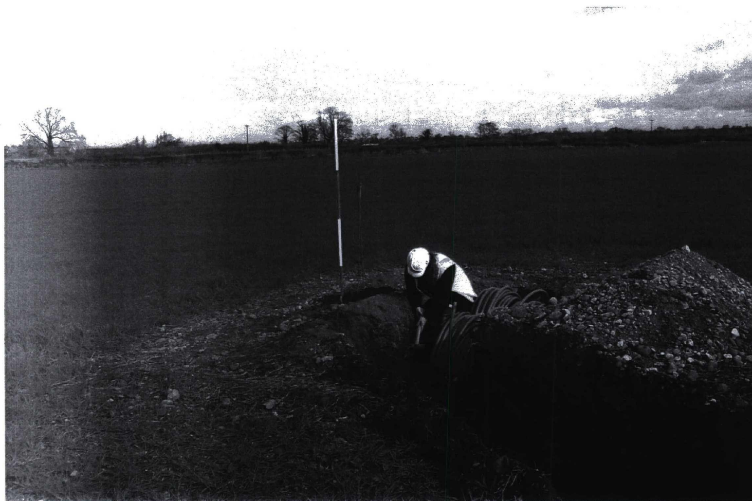
Plate 13. Placing of aluminium marker at junction of Trench 1 and previous excavated pipe trench. Facing north.
