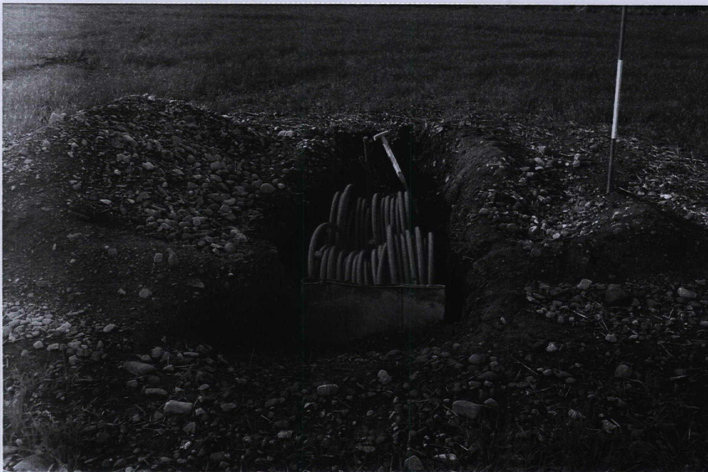
Plate 3. Open junction trench with water pipes in situ. Facing South-west.
