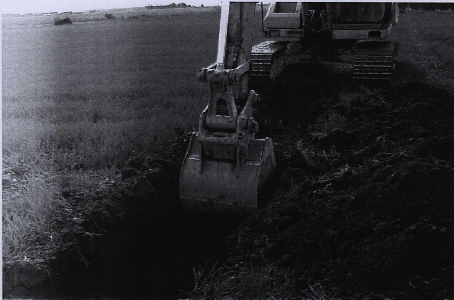
Plate 11. Trench 1 under excavation, removal of the subsoil. Facing south-east.
