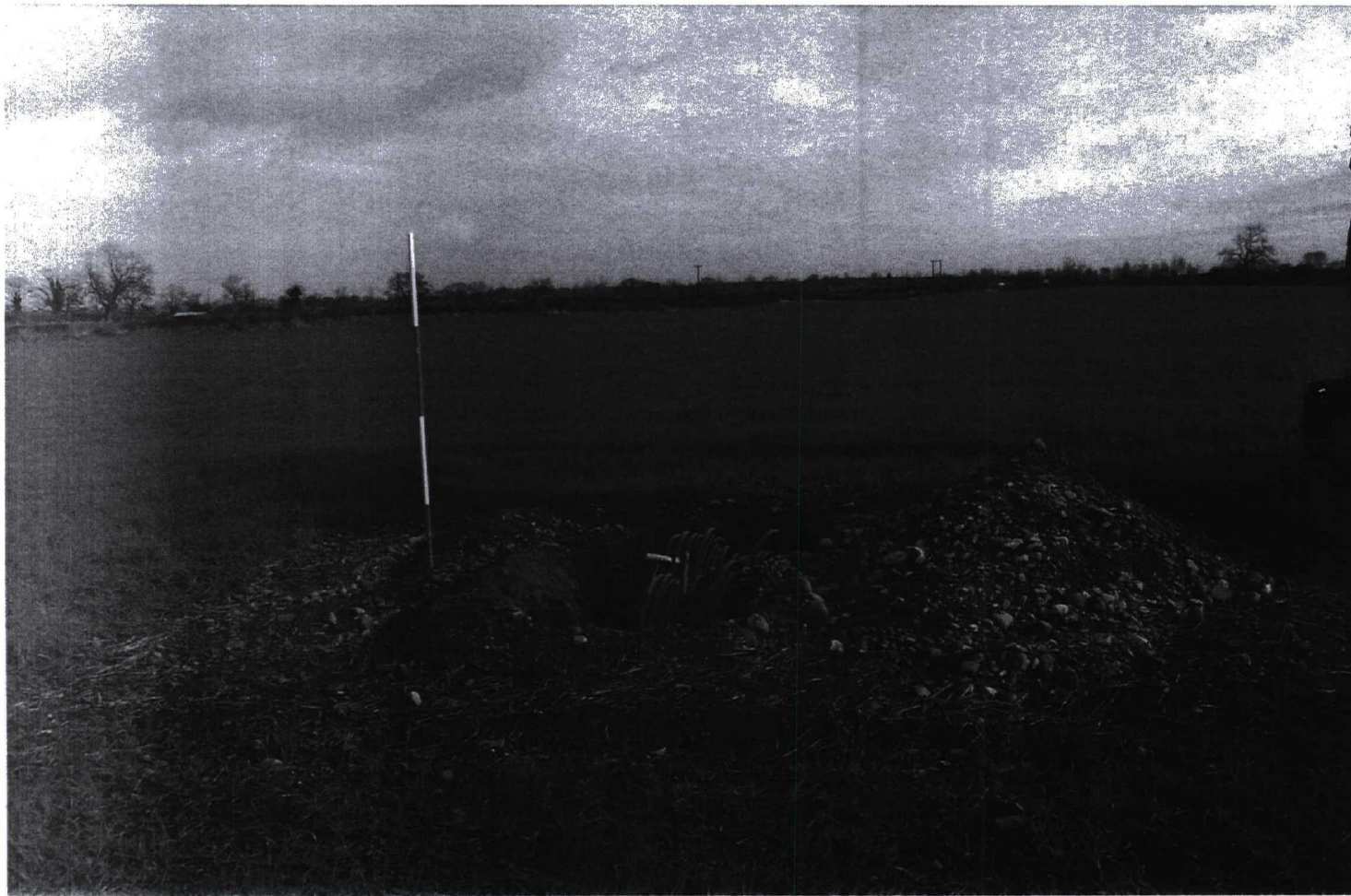
Plate 1. Location of junction with previous pipe trench excavation. Facing north-east.
