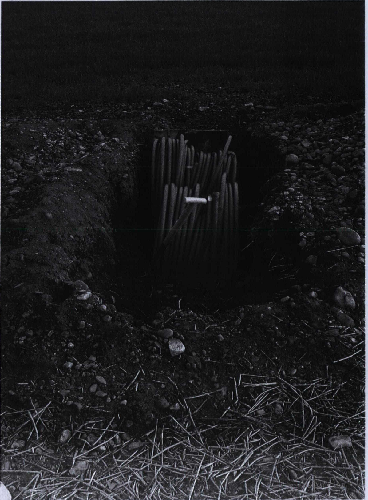
Plate 2. Open junction trench with water pipes in situ. Facing north-east.
