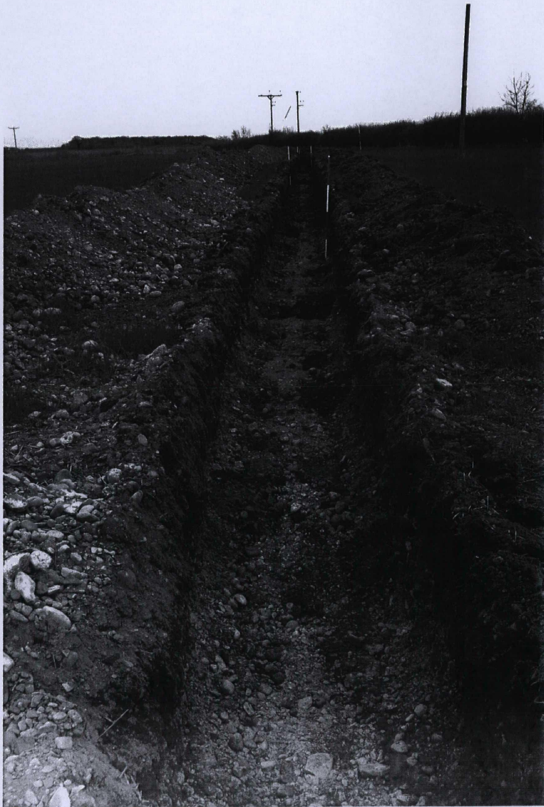
Plate 54. Completed excavation of Trench 1. Facing south-east.
