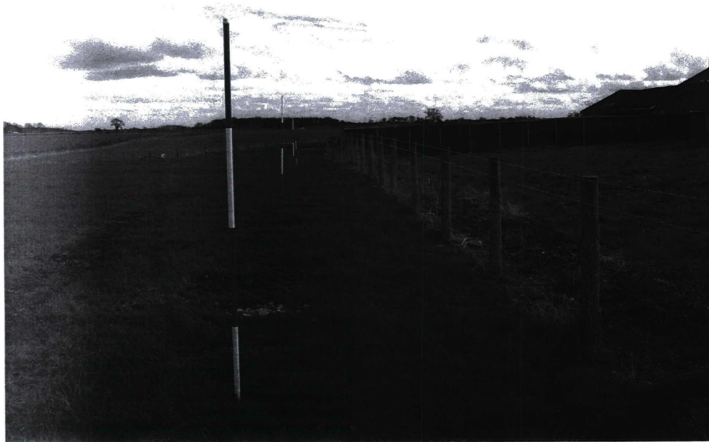
Plate 46. Alignment of Trench 3 pipe trench, prior to excavation. Facing south-east.
