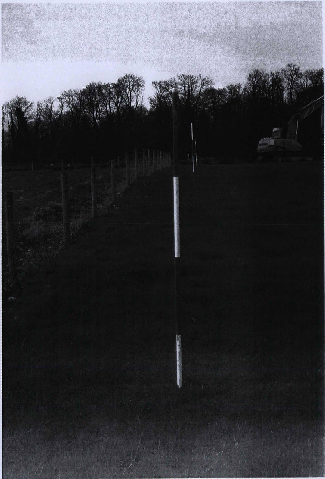
Plate 47. Alignment of Trench 3 pipe trench, prior to excavation. Facing north-west.
