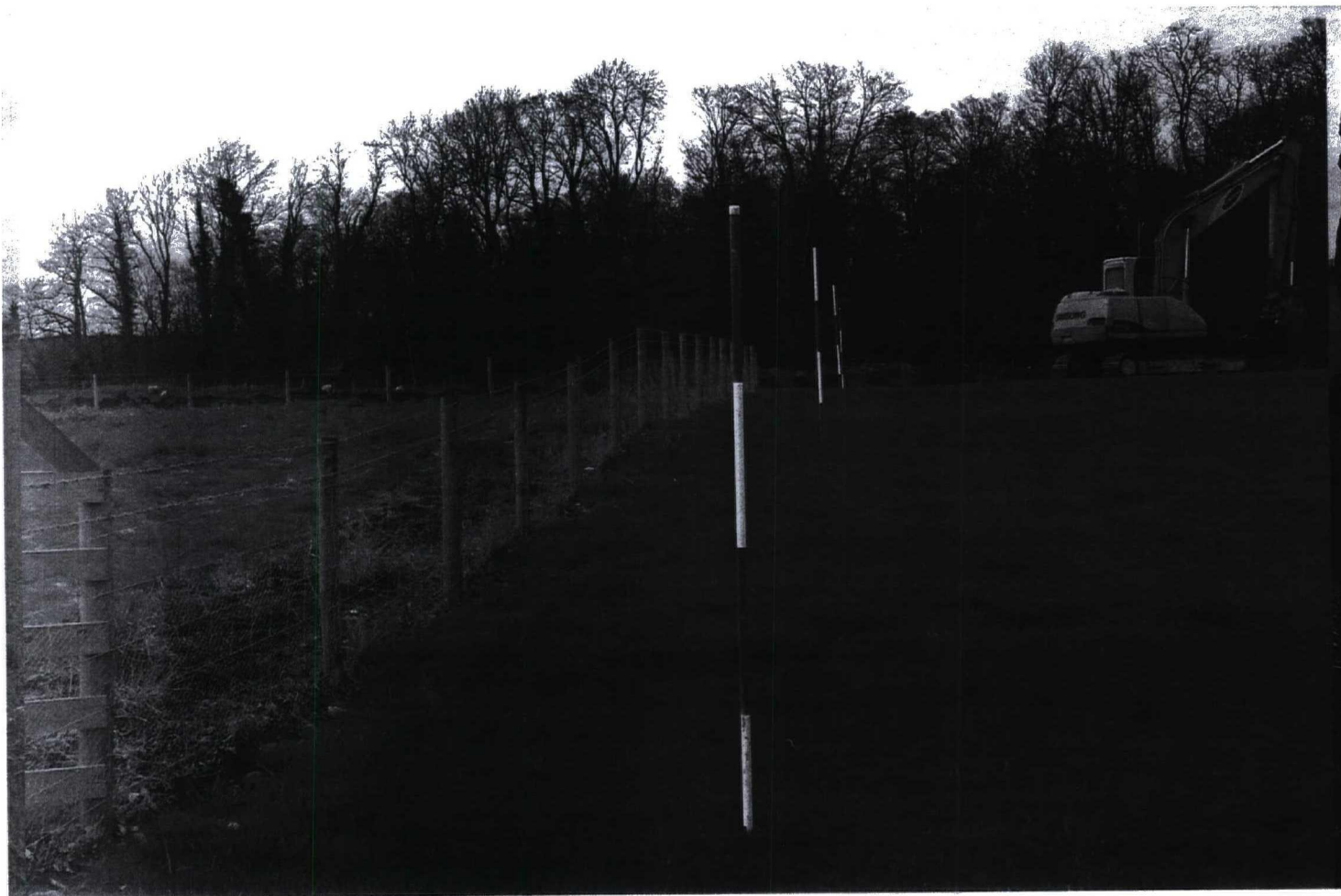
Plate 48. Alignment of Trench 3 pipe trench, prior to excavation. Facing North-west.
