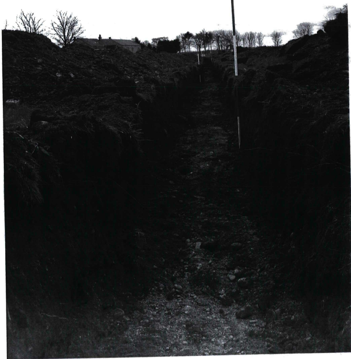
Plate 41. Completed excavation of Trench 2. Facing south-west.
