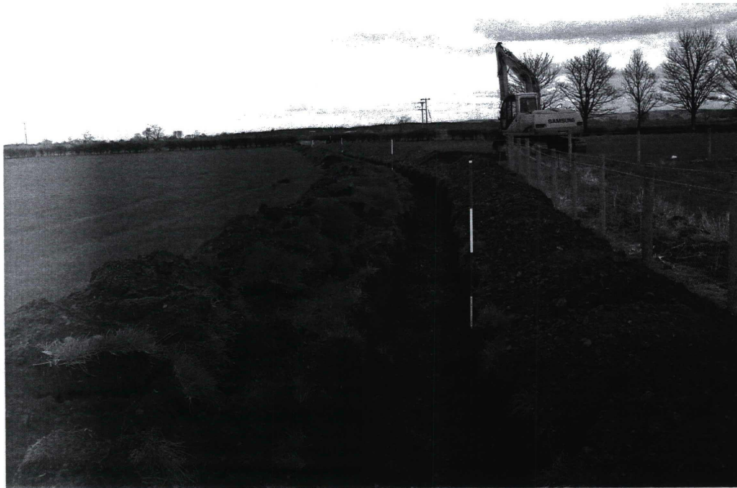
Plate 43. Completed excavation of Trench 2. Facing north-east.
