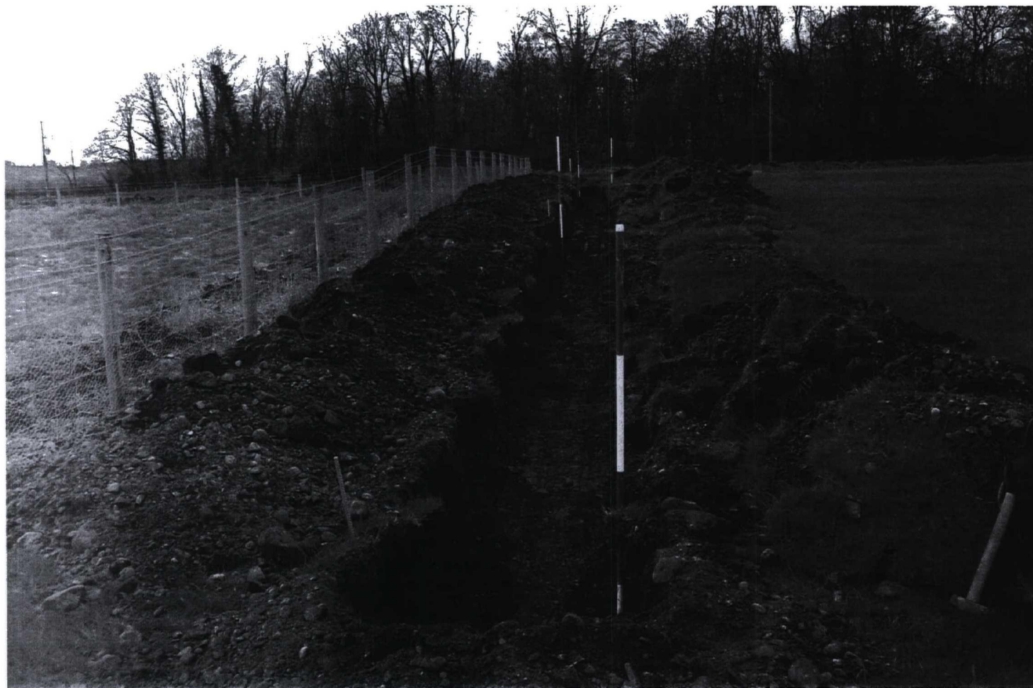
Plate 51. Completed excavation of Trench 3. Facing north-west.
