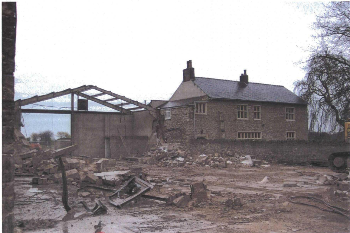
Plate 26. Demolition of Drying Shed, Facing East
