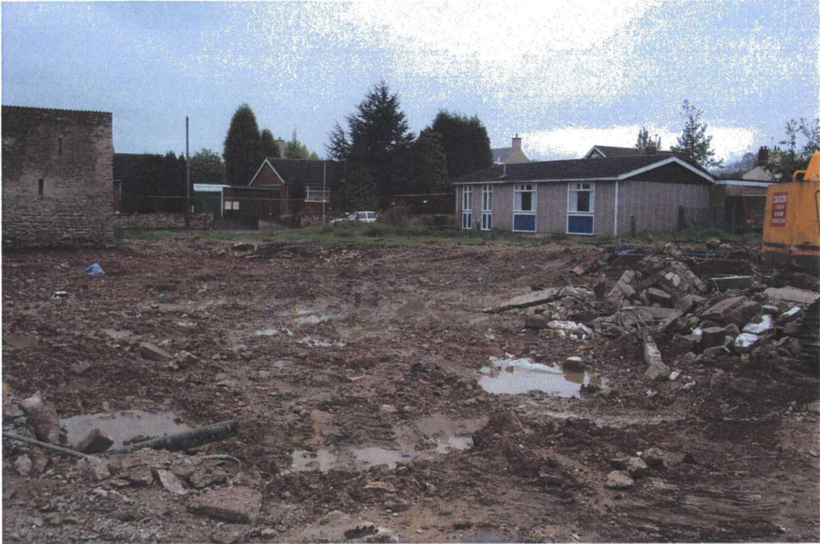
Plate 27. Demolition of Drying Shed, with Barn in Background, Facing East
