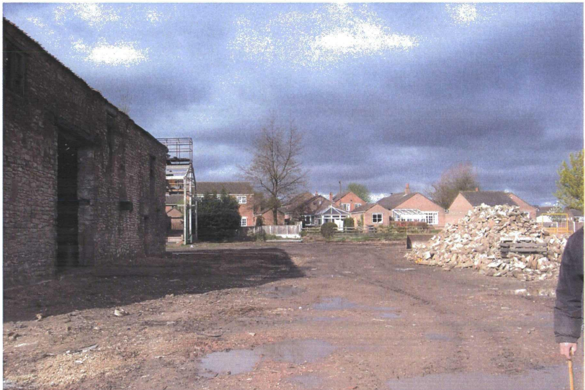
Plate 8. View of Barn and House, Facing South
