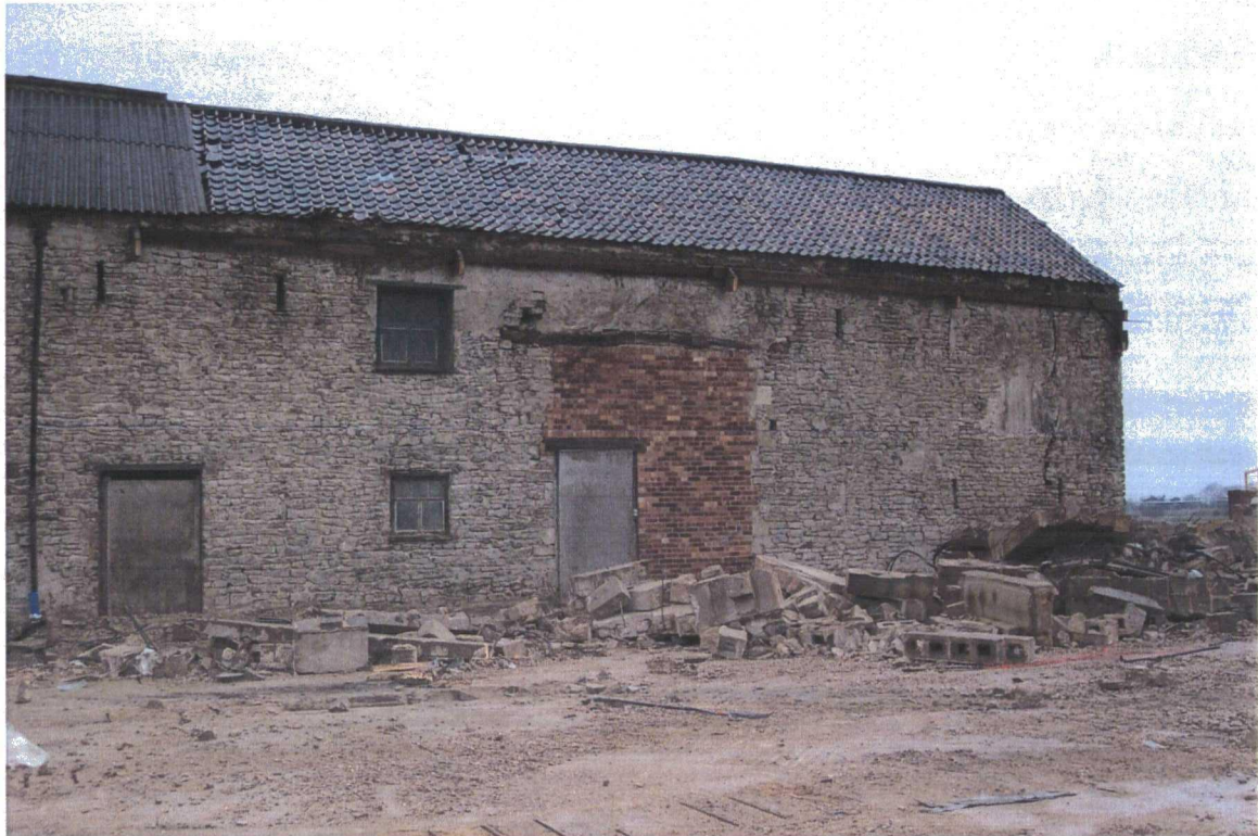
Plate 24. Barn Exterior after Shed Demolition, Facing North
