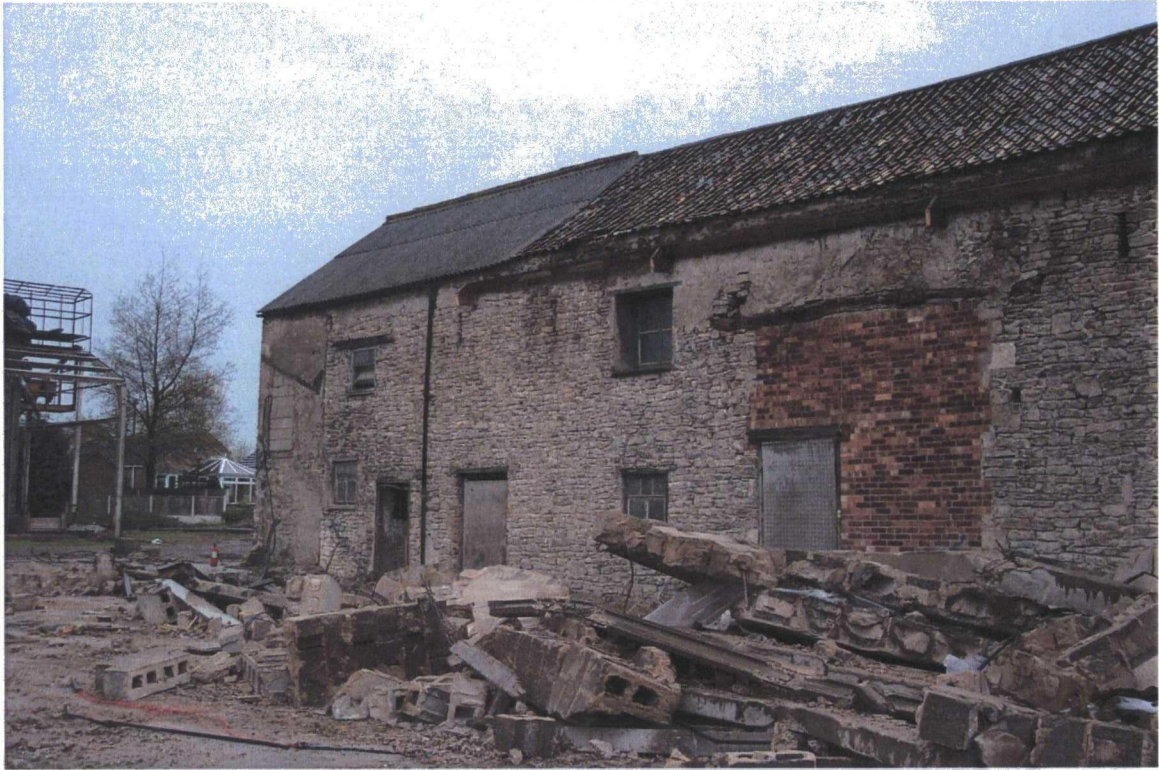
Plate 23. Barn Exterior after Shed Demolition, Facing North West
