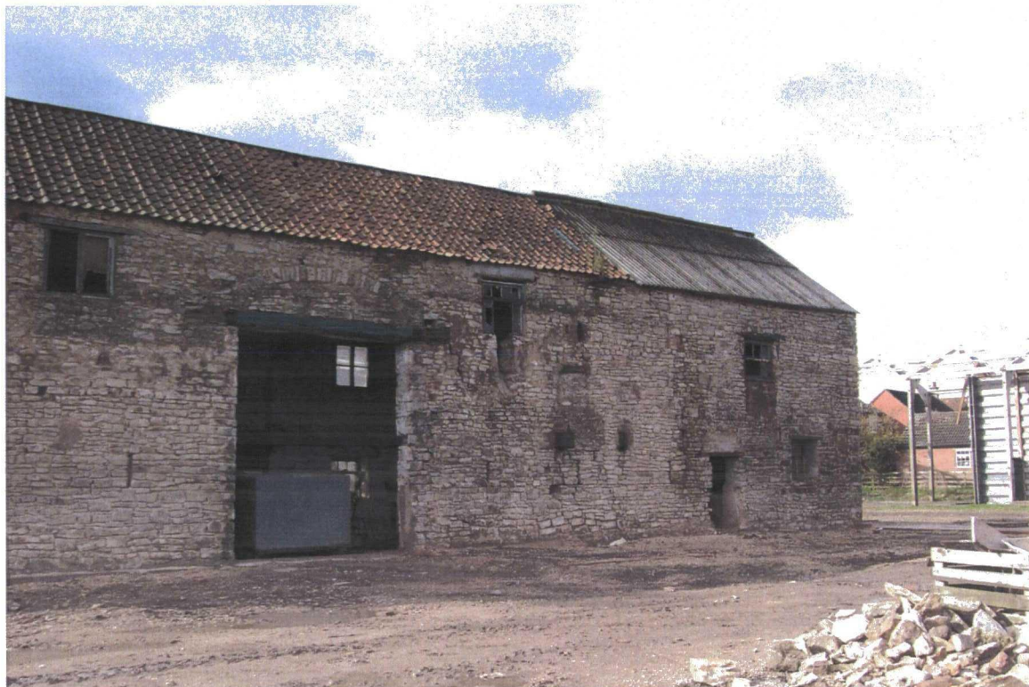
Plate 4. View of Site and Dutch Barn, Facing East
