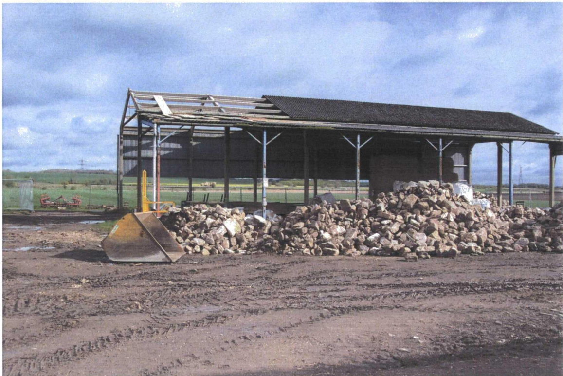
Plate 2. View of Site and Dutch Barn, Facing North
