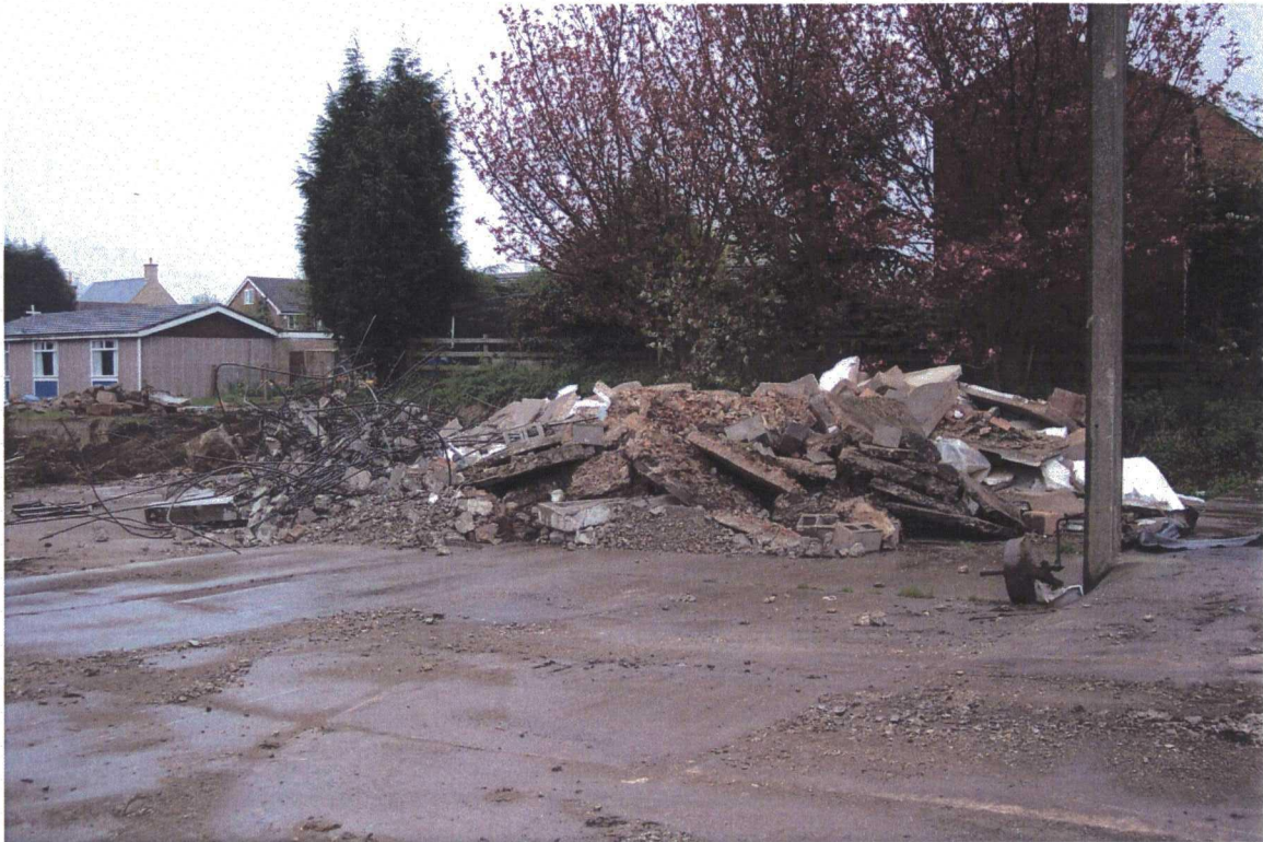
Plate 19. Site Demolition, Facing South West
