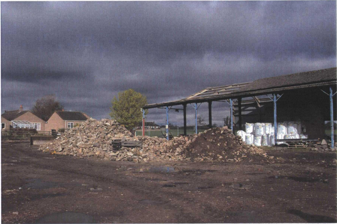
Plate 9. View of Barn and Site, Facing West
