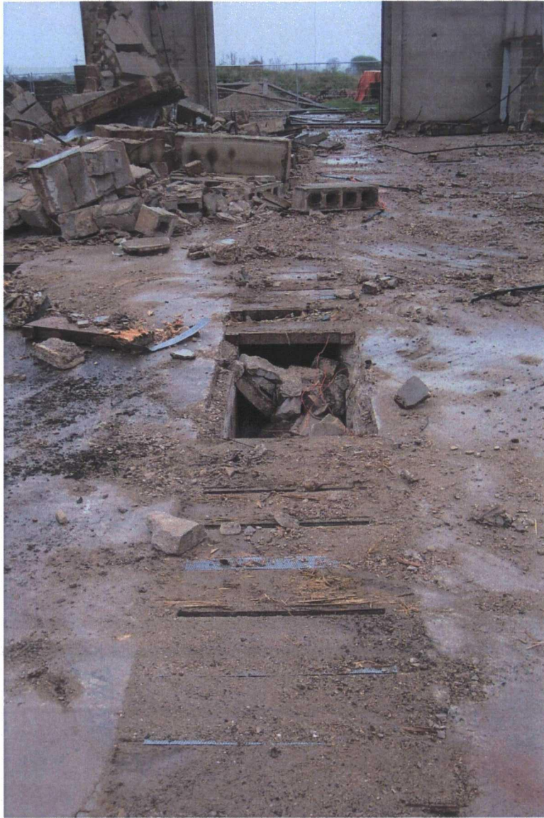
Plate 25. Foundations of Drying Shed, Facing East
