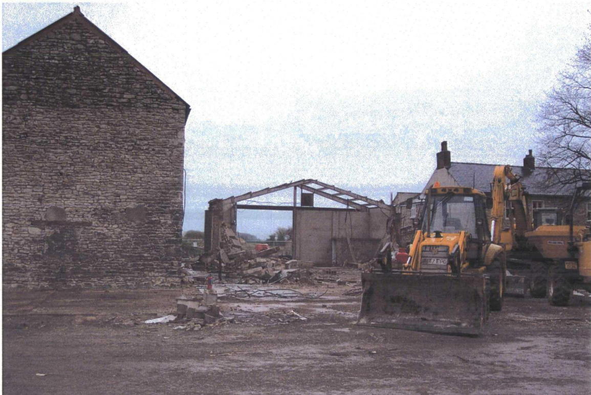
Plate 20. Barn and Demolition of Drying Shed, Facing West
