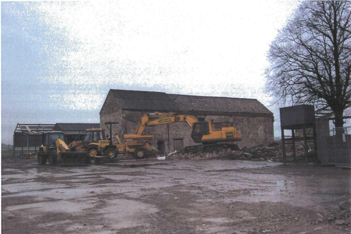
Plate 28. View of Access Road after Demolition, Facing South West
