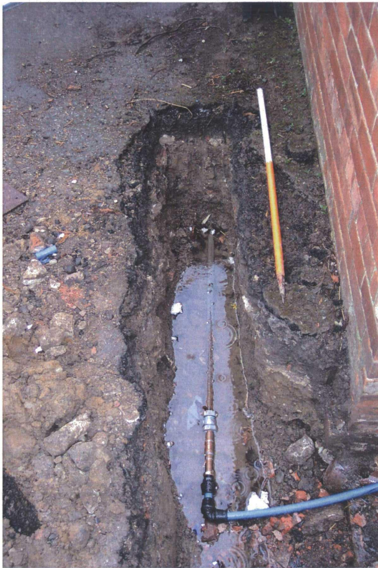
Plate 17. Drain Excavation, Facing South
