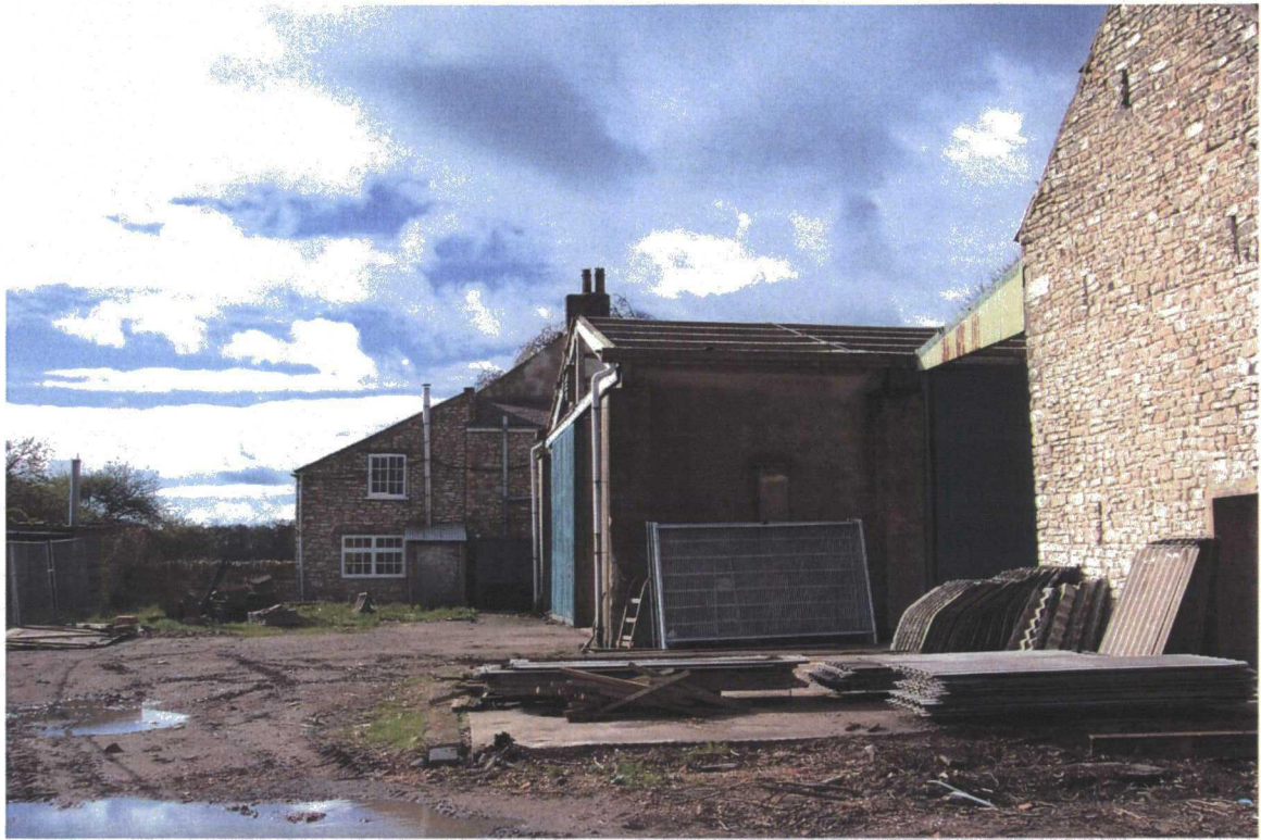
Plate 7. View of Barn, Facing South West
