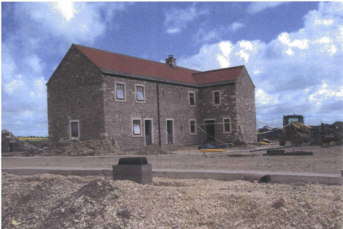
Plate 56. View of Barn, Facing North East
