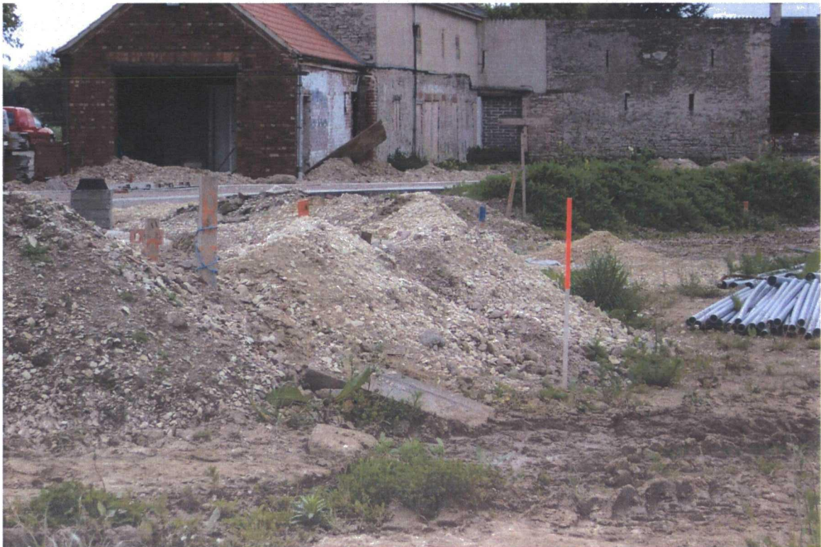
Plate 52. View of Site - Road Alignment, Facing South
