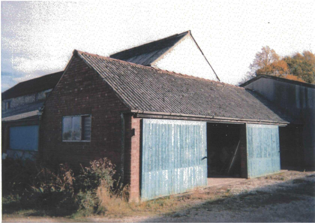
Plate 68. External View of Stone Barn with Brick and Corrugated Iron Additions
