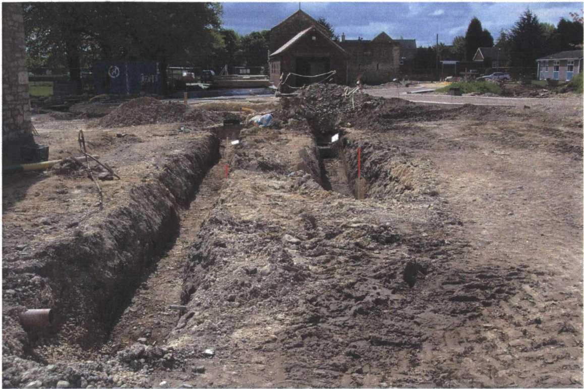
Plate 59. Drain Runs, Facing South
