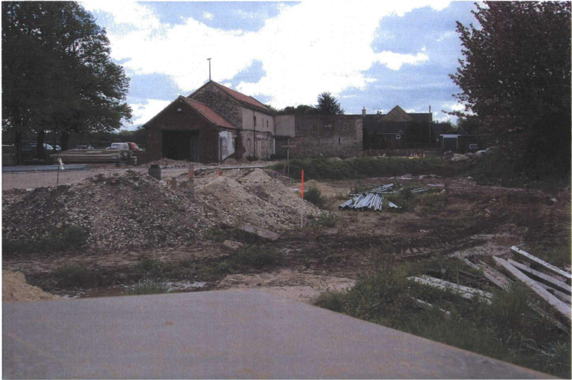
Plate 51. View of Site - Road Alignment, Facing South
