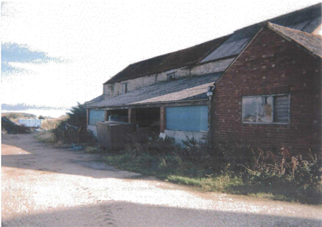
Plate 69. External View of Stone Barn with Brick and Corrugated Iron Additions
