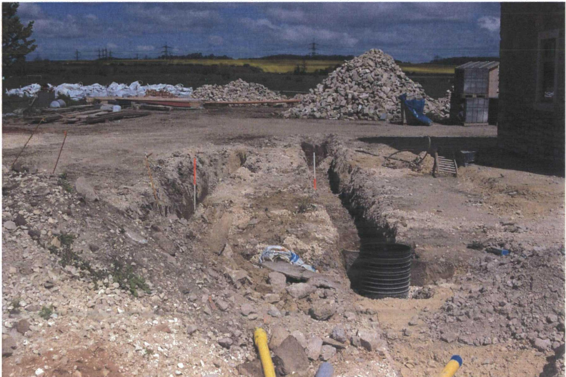
Plate 60. Drain Runs, Facing North
