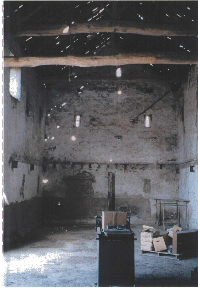
Plate 83. Internal View of Old Barn
