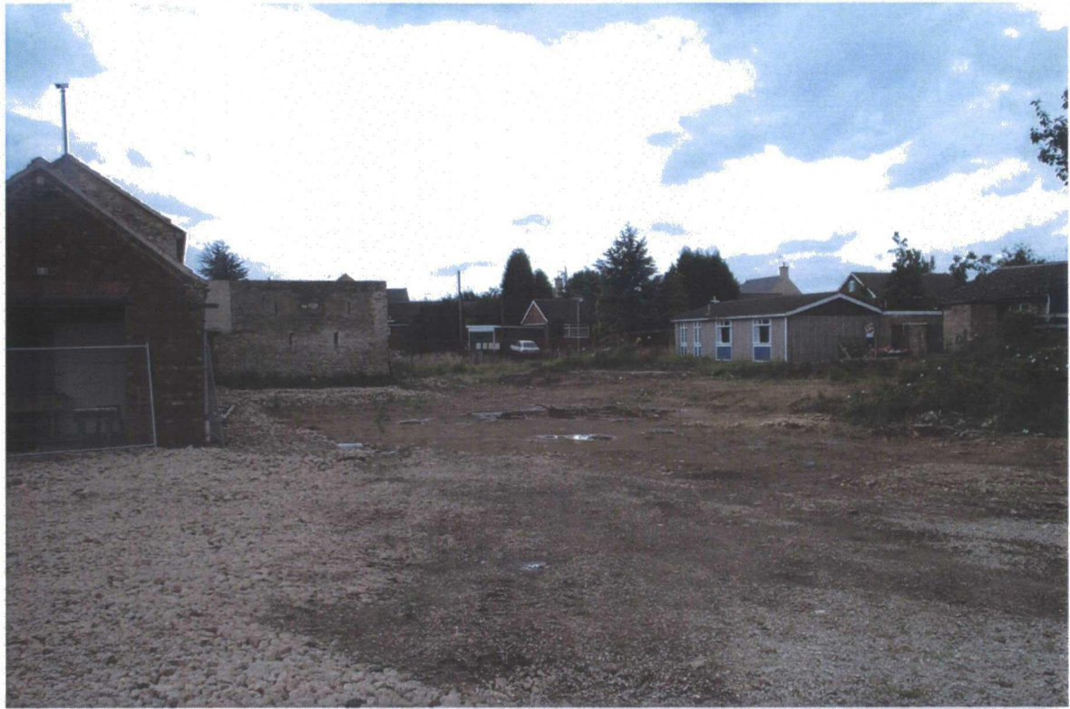
Plate 94. External View of Old Barn after Demolition of Brick and Corrugated Iron Structures
