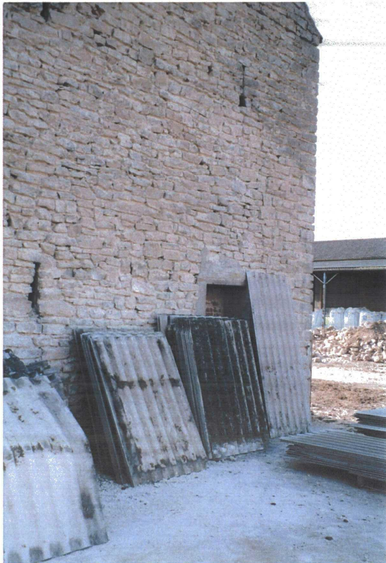
Plate 81. External View of Old Barn after Demolition of Brick and Corrugated Iron Structures
