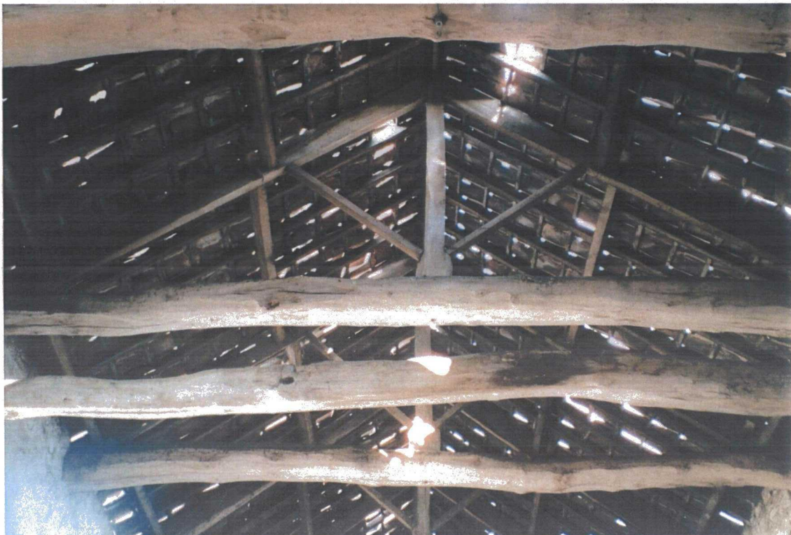
Plate 85. Internal View of Old Barn
