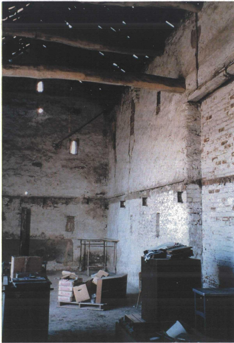
Plate 84. Internal View of Old Barn
