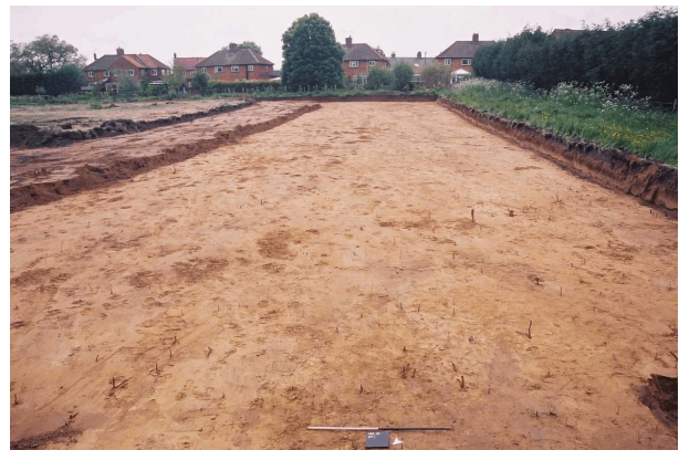
Plate 5 Subsoil in northern spur (looking south)
