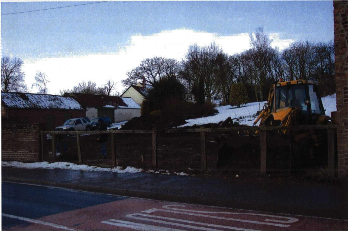
Plate 1. View of Site. Facing South West
