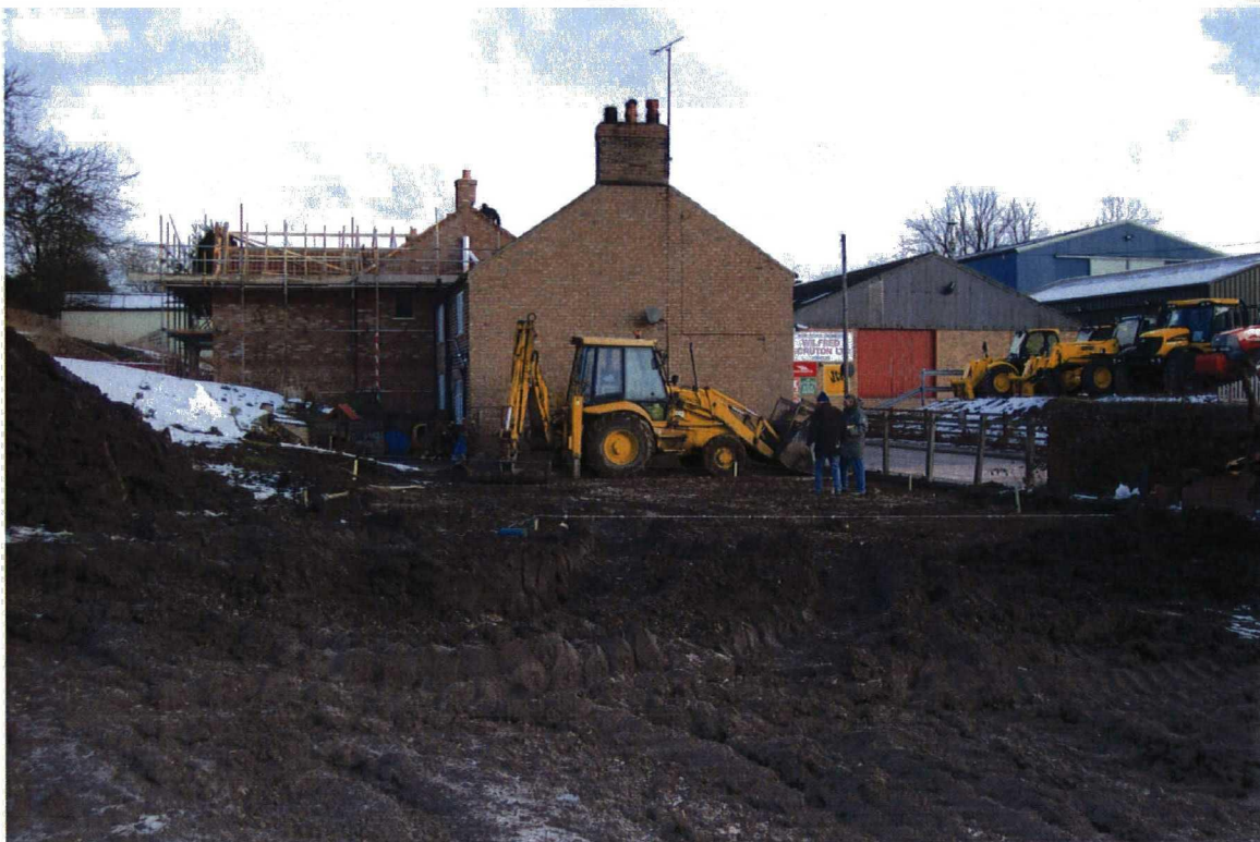
Plate 2. View of Site. Facing North
