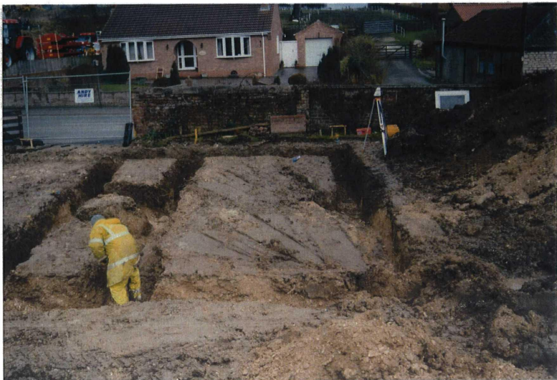
Plate 4. View of Footings. Facing East
