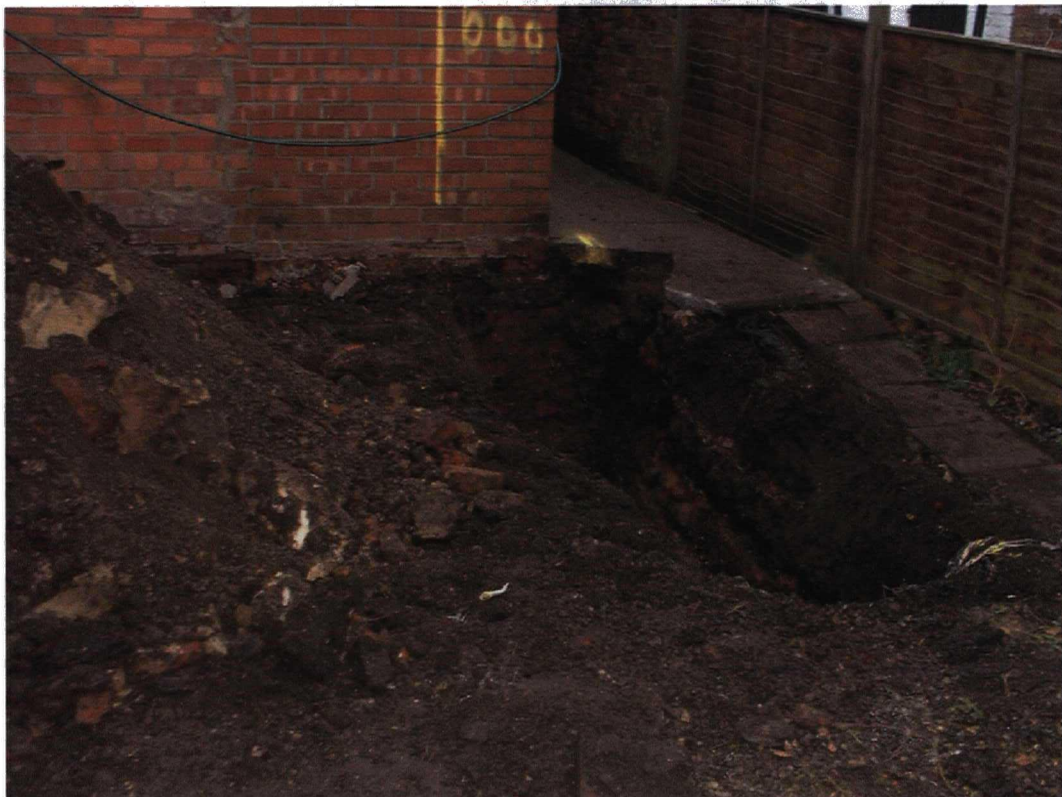
Plate 2. Excavation of Foundation, Facing South
