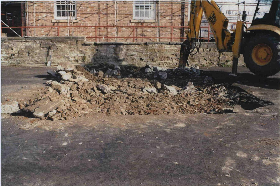
Plate 1. General view of excavation. Facing Northeast
