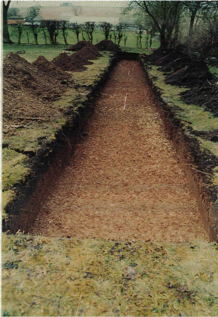
Plate 1. Trench 1. General Shot. Facing North.
