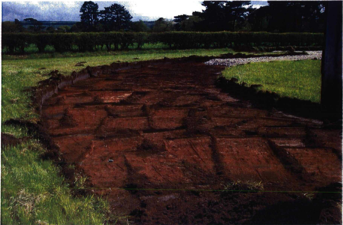
Plate 3. Excavated Road Section. Facing South East
