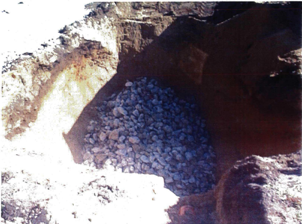
Plate 12. Soakaway Being Back-Filled, Facing East
