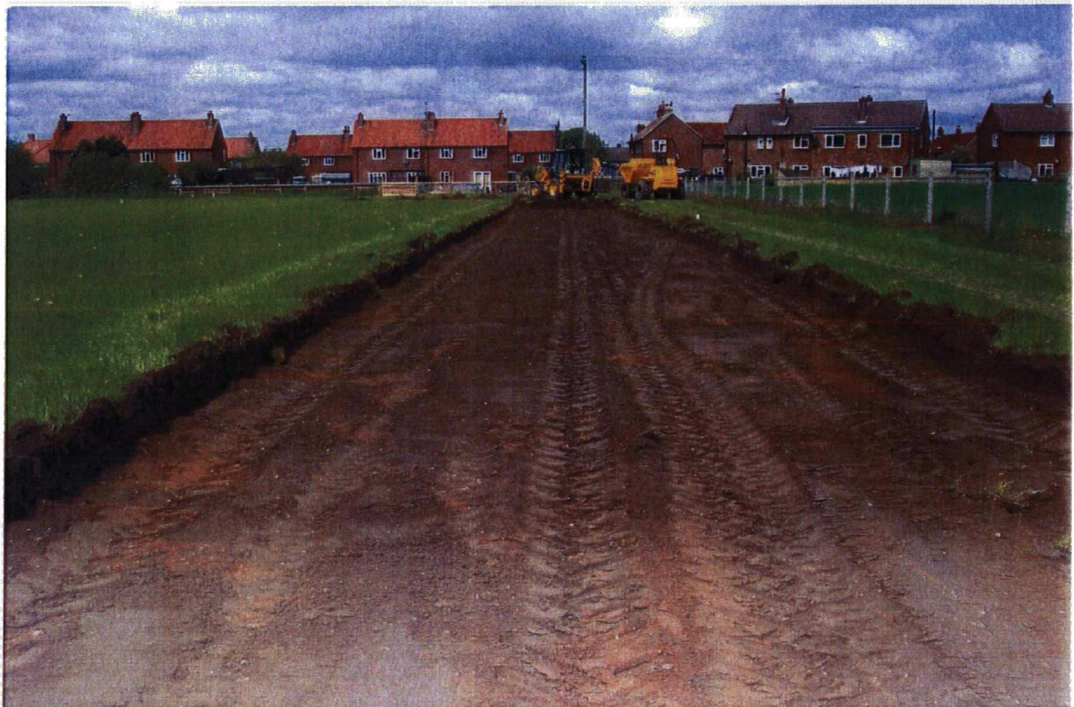
Plate 4. Excavated Road Section. Facing North West
