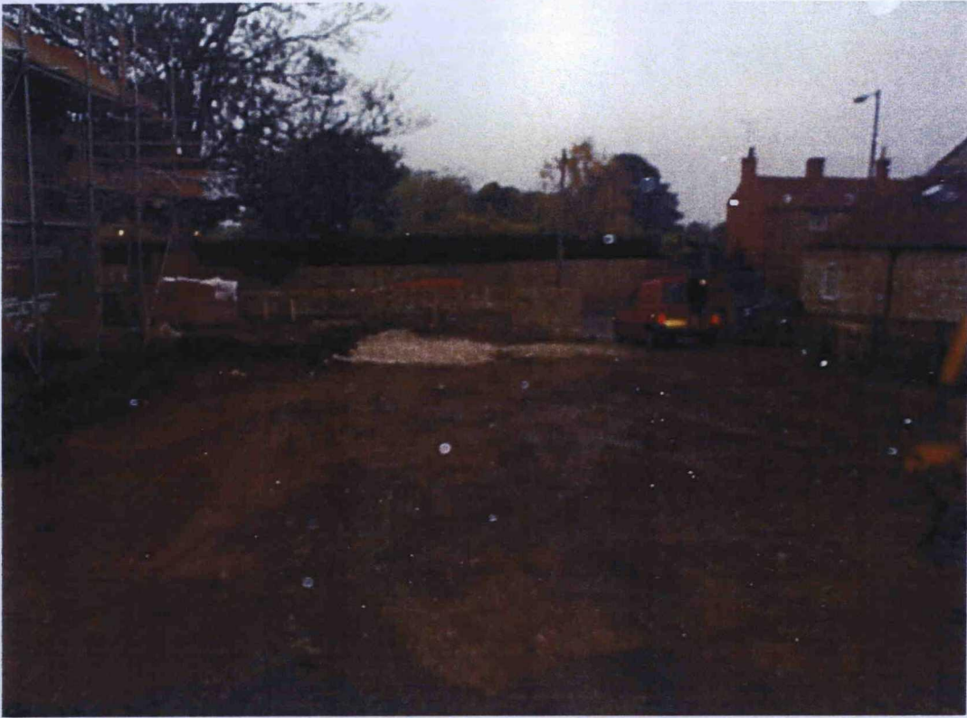
Plate 3. Prior to Excavation of Foundation Trenches. Facing North East
