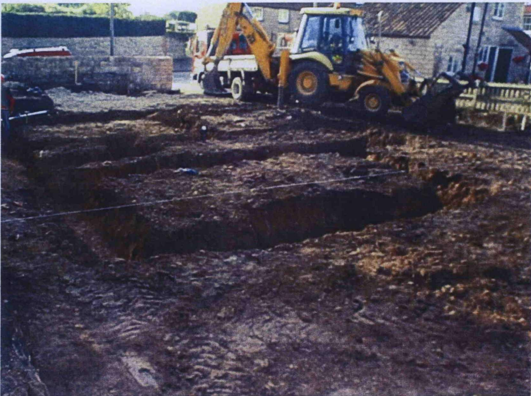
Plate 4. Post-Excavation Photo of Foundation Trench. Facing South East
