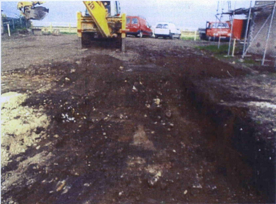
Plate 1. Overall Photo of Phase 1 Stripping. Facing East
