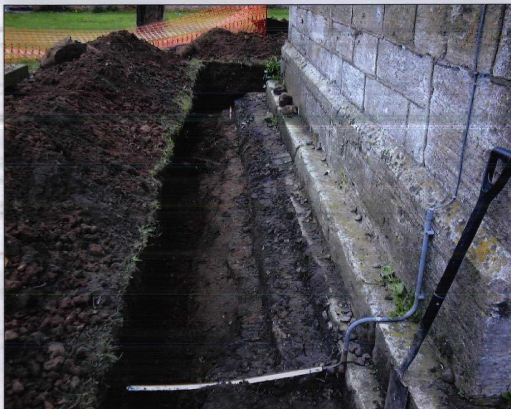
Plate 5. Exposed foundations of the west tower, Trench 1, view north.
