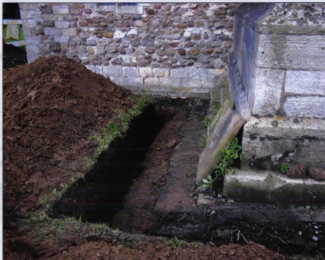
Plate 6. Trench 1, view east towards north transept. (Scale of 0.5m).
