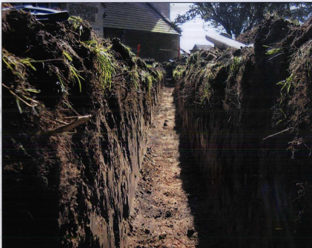
Plate 2. Trench 1, view south towards Long Marston church.
