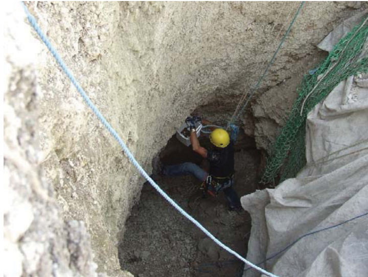
Plate 23: Abseiling down the side of the collapsed area to take a sample (photo number 661-6461-27)
