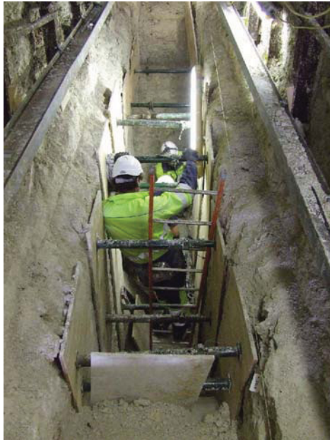
Plate 10: The ditch excavation below the tunnel floor (photo number 661-6282-01)
