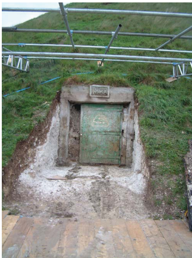
Plate 25: The portal area after being exposed (photo number 661-6004-04)
