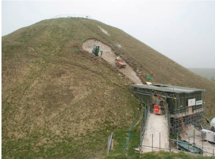
Plate 18: The hillside Watching Brief (Photo number 661-6862-07)
