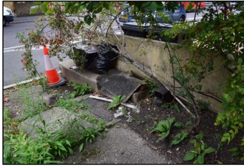
Photo 2: Manhole cover in the front yard
