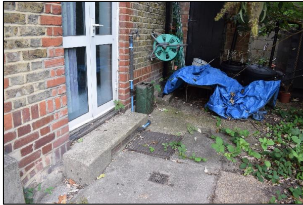
Photo 5: Manhole covers at the rear of the building
