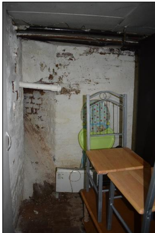
Photo 6: View within the existing cellar
