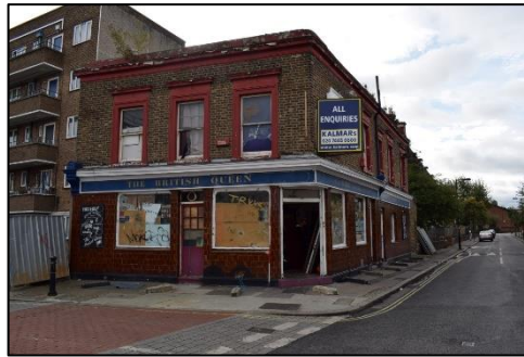
Photo 1: The north & west elevations of the British Queen Public House (scale 2m)
