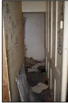
Photo 13: View of the 1 st floor landing, from the north
