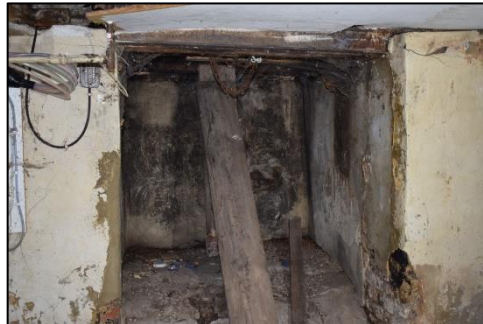
Photo 17: The interior of the basement dray chute hatch
