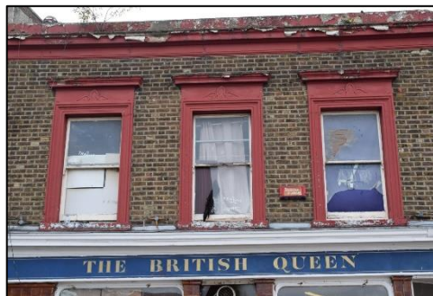
Photo 6: 1 st floor windows with moulded stucco surrounds & cornice
