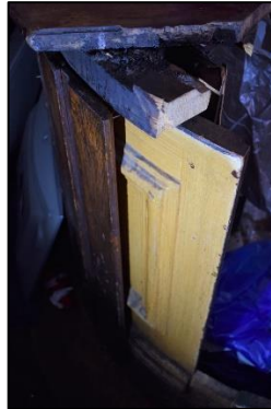
Photo 11: Earlier bar panelling exposed beneath later panelling
