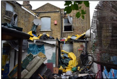
Photo 8: Rear elevation from the service yard
