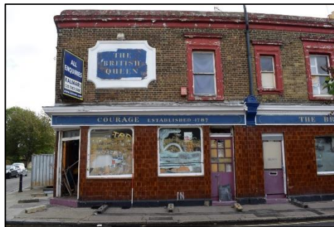
Photo 4: North end of the west elevation (early door centre)
