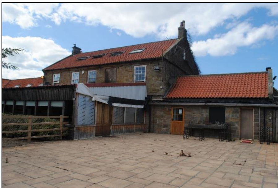
Photo 4. Cross Butts [AB 1] south elevation; view north/northwest
