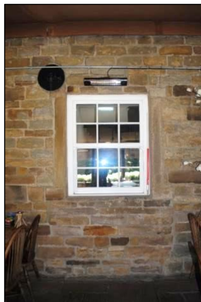
Photo 65. Window inserted into a former doorway; view N
