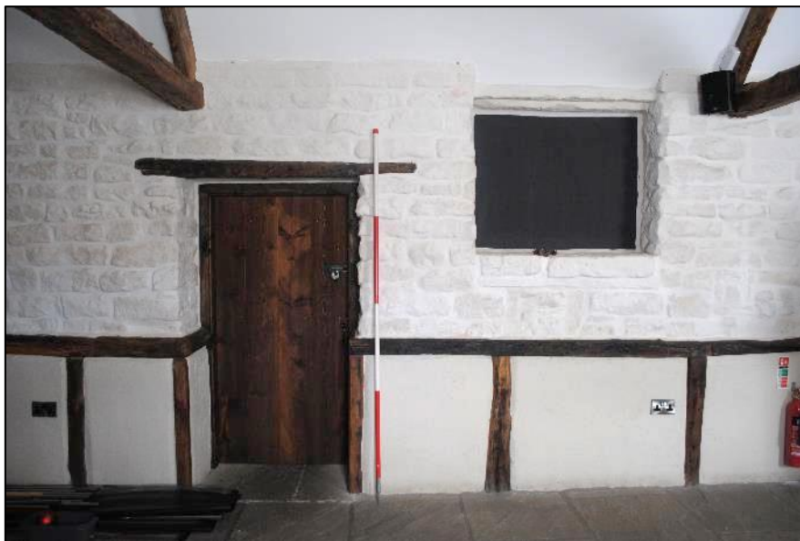
Photo 28. Room G4 – east wall; northern doorway and blocked window
