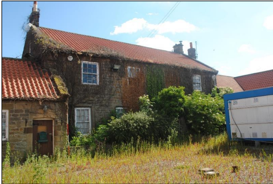
Photo 2. North elevation of Cross Butts Farmhouse [AB 1]
