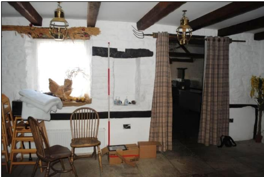
Photo 71. Cottage [AB 3] north wall; view NE
