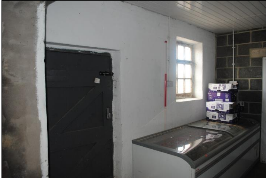
Photo 87. Northern end of the barn; interior; view NE
