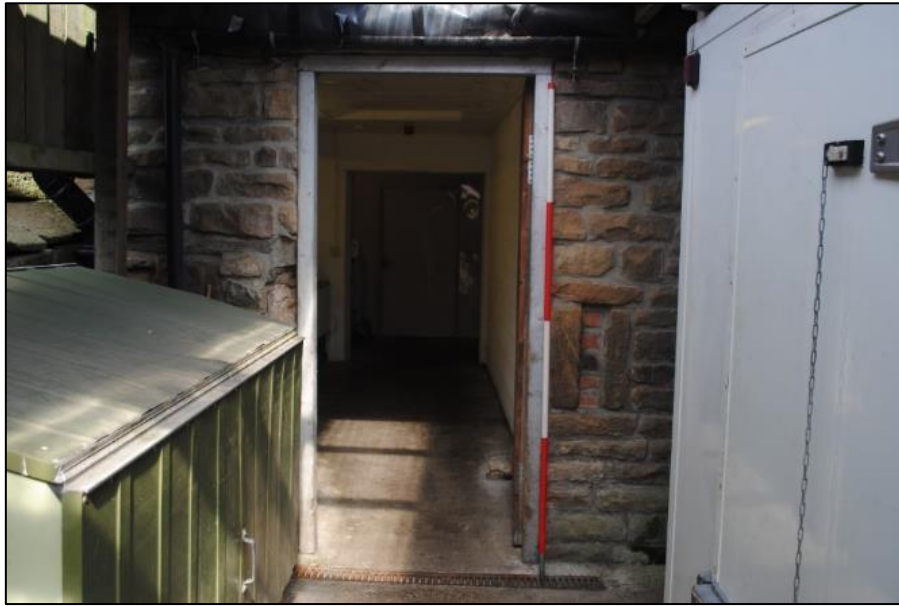
Photo 24. AB 2 west wall, north doorway
