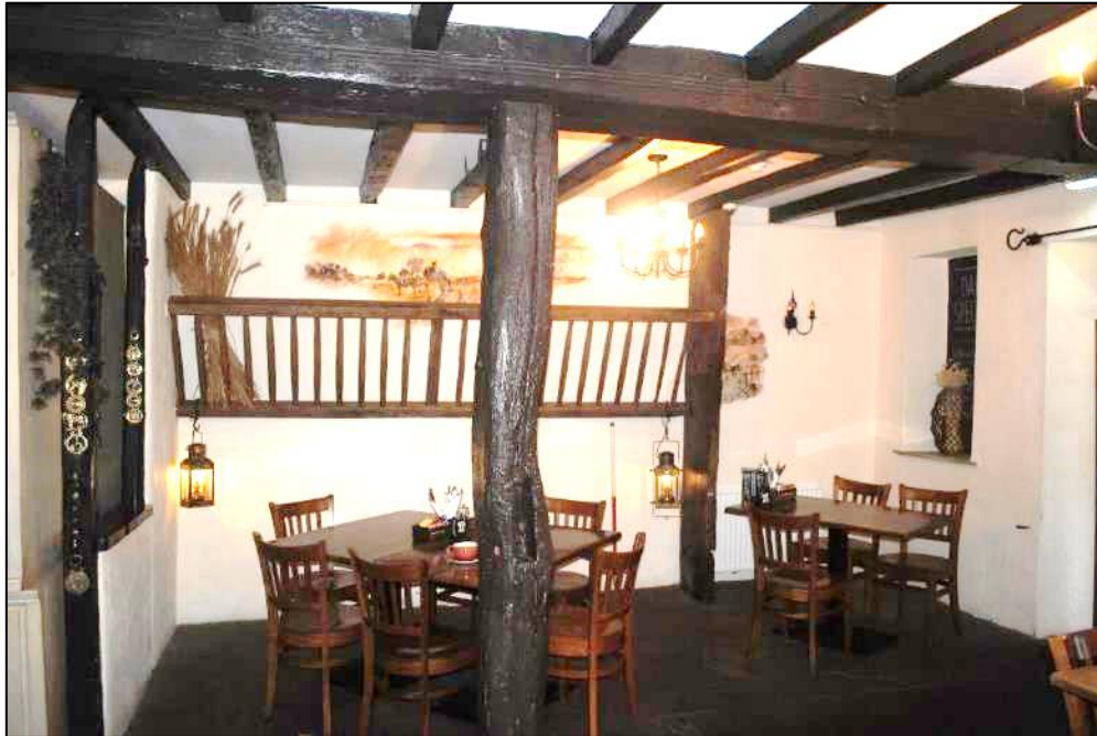
Photo 8. AB1 – G2; central partition wall between G1 and G2; view east
