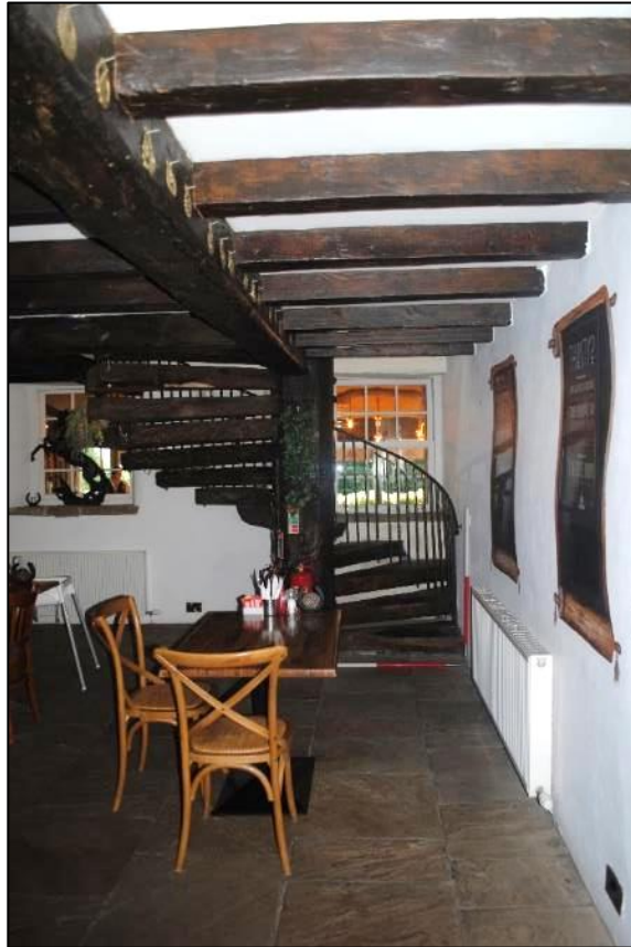
Photo 7. AB1 – G1; modern spiral staircase from ground to first floor; view south
