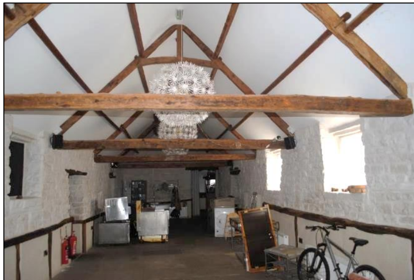
Photo 30. Room G4 – south gable; view south
