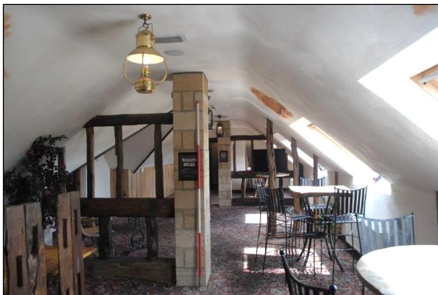
Photo 53. Room R3; view east into Room R4
