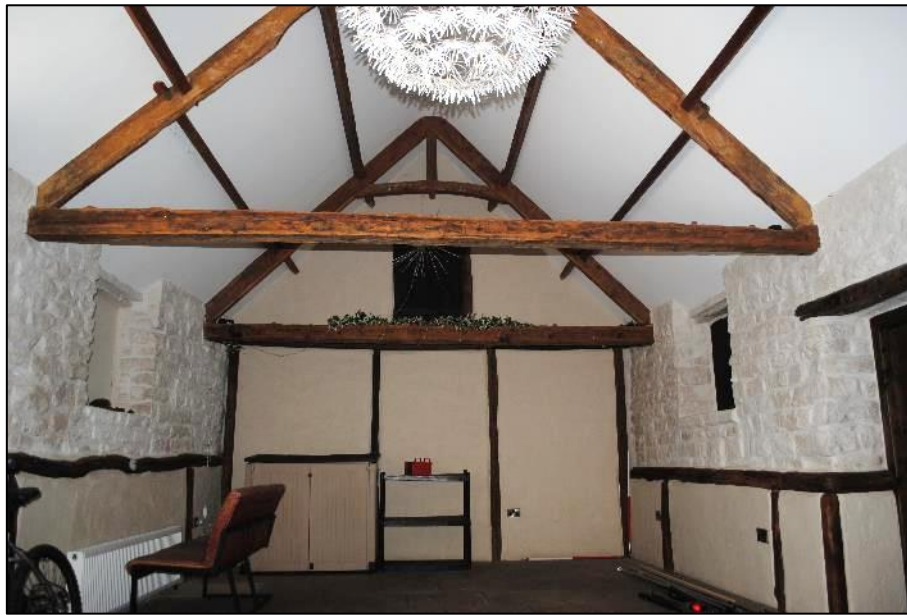
Photo 27. Room G4 – north wall; view north
