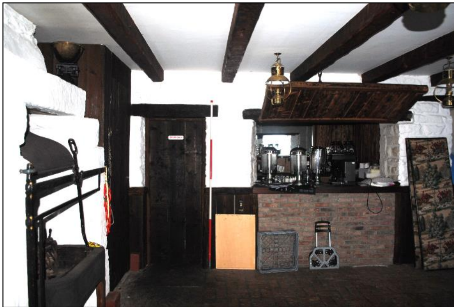
Photo 73. Cottage [AB 3] south wall; view south
