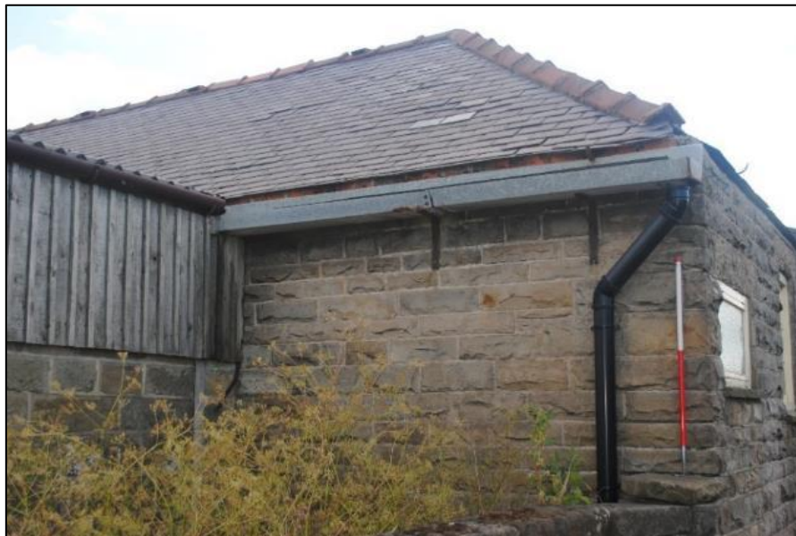
Photo 80. NE corner of the Barn; view SE
