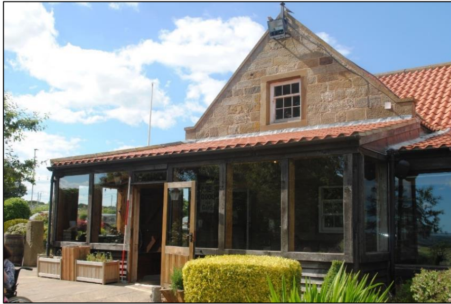
Photo 56. Structure E1; view NW from the beer garden
