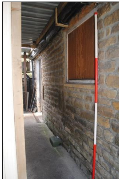
Photo 23. AB 2 west wall; view NE
