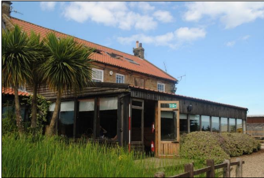
Photo 58. Sun Terrace (S1); view NE
