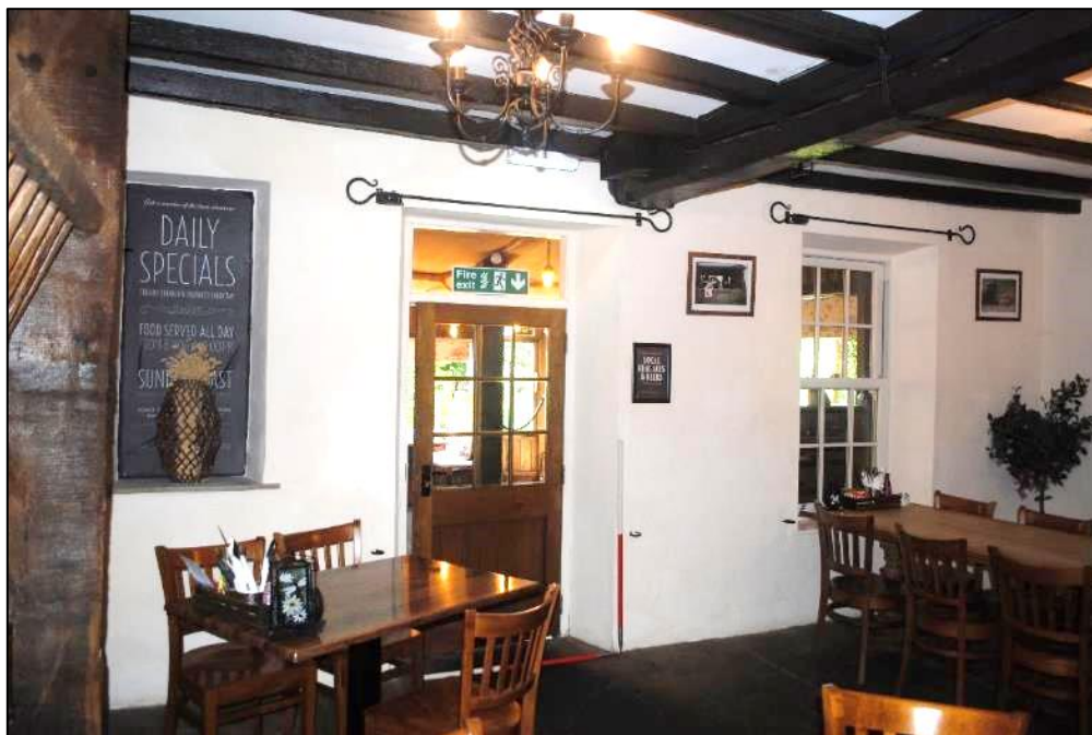
Photo 9. AB1 – G2; south wall; the current doorway to the Sun Terrace and enlarged window
