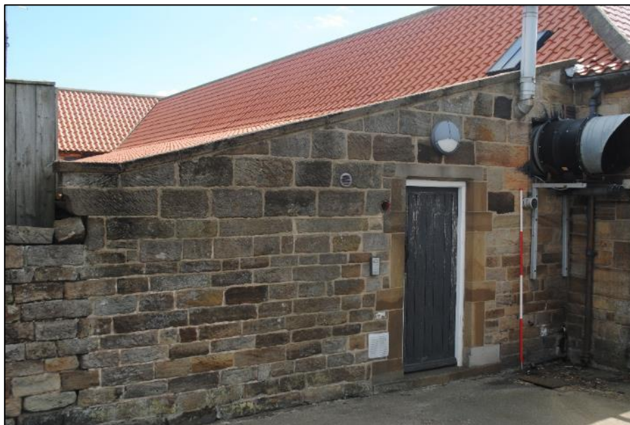
Photo 35. North wall of the Kitchen extension (K1); view SW
