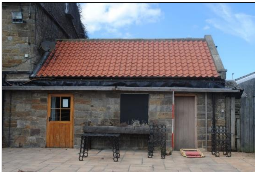
Photo 68. The modern south elevation of the Cottage [AB3]
