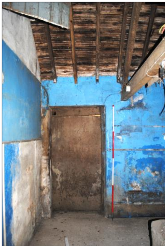
Photo 86. Blocked doorway leading to the neighbouring property
