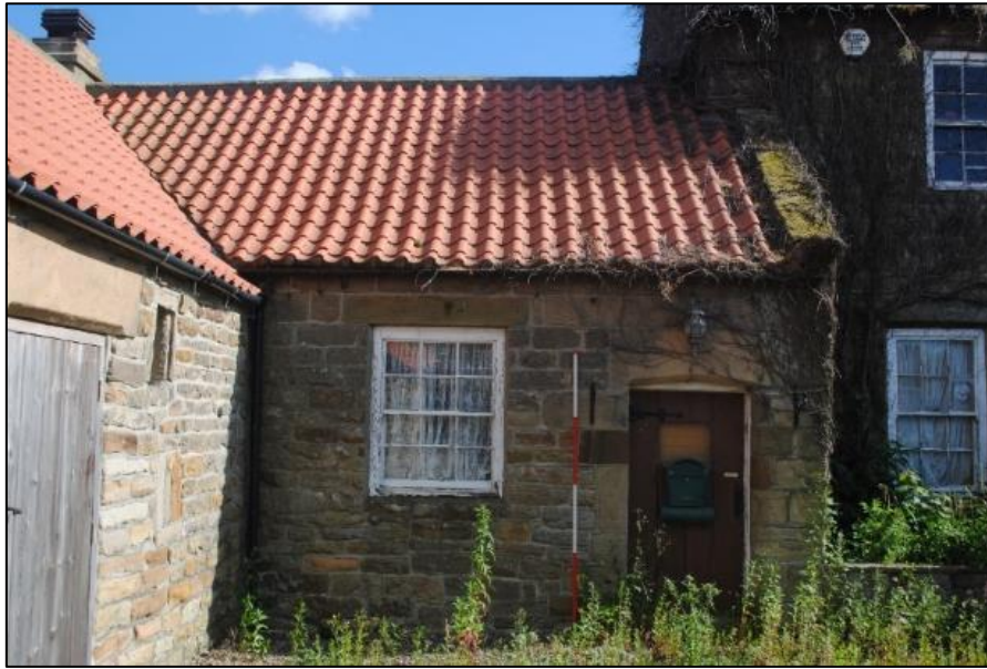
Photo 67. North elevation of the Cottage [AB 3]
