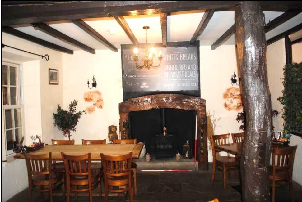
Photo 10. AB1- G2; west wall; modern fireplace; with additional metal flue
