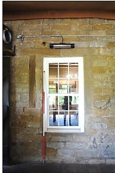
Photo 66. Sash-window replacing an earlier square opening; view N
