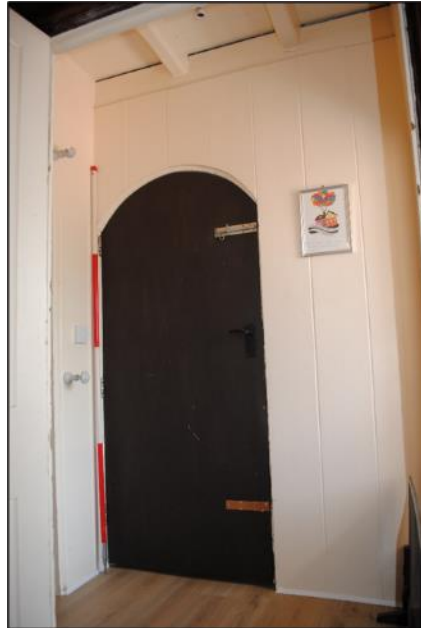
Photo 16. First Floor stairwell; door leading the kitchen; view E/NE
