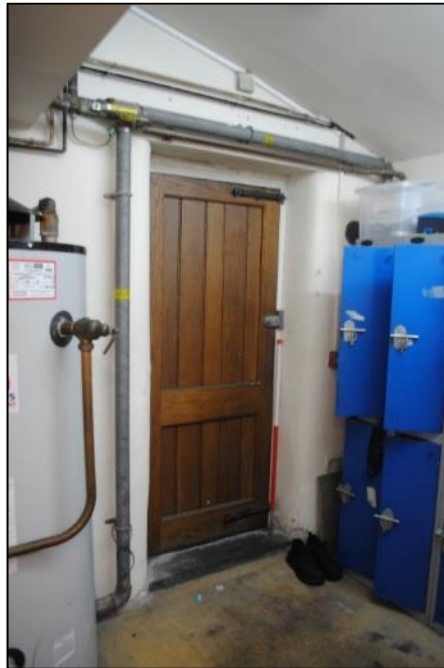
Photo 43. Kitchen staff changing area; view N/NE
