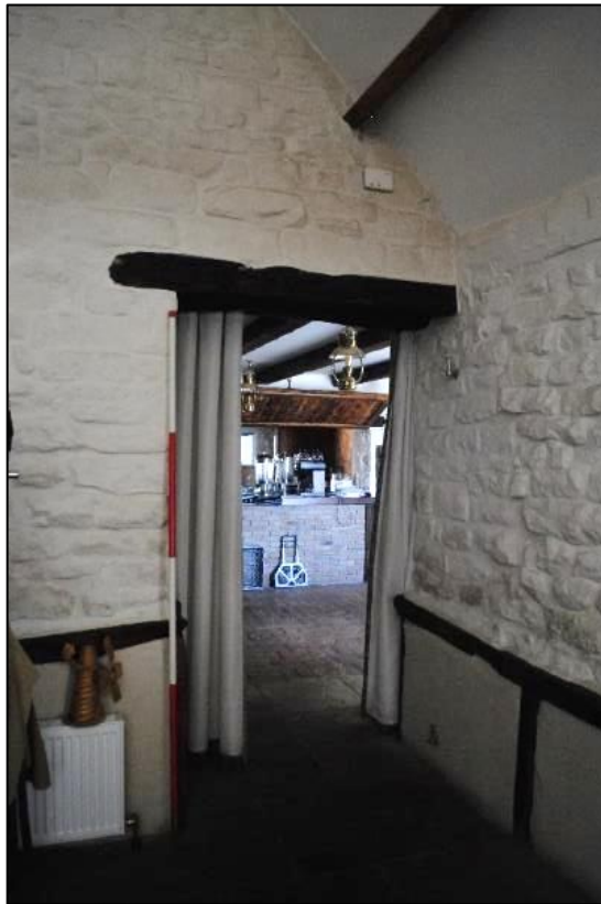
Photo 31. Doorway from G4 into the Cottage [AB 3]; view S/SW
