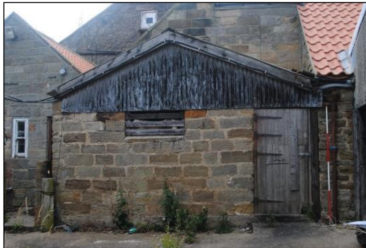
Photo 76. East wall of the Outhouse
