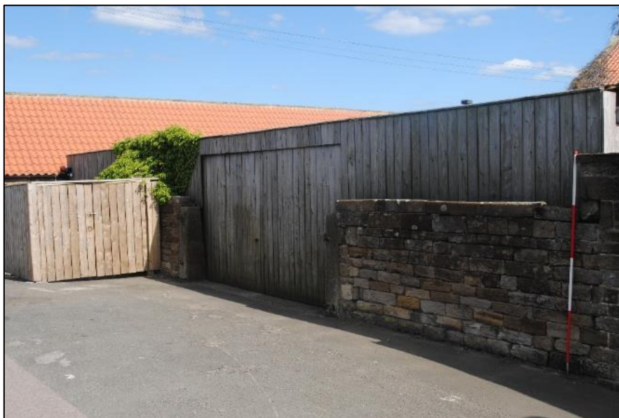
Photo 88. Farmyard from the Guisborough Road, 2022; view SE
