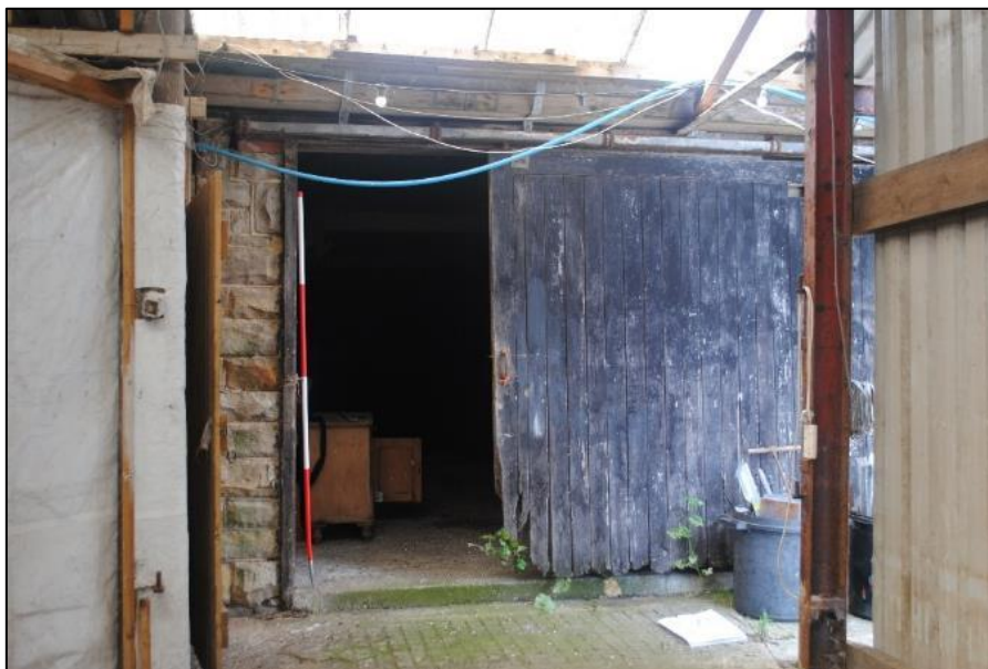
Photo 82. Barn, south elevation; large sliding cart-door; view N/NE
