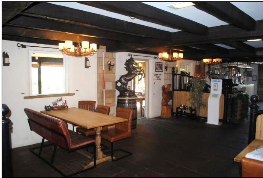
Photo 50. View SW within Room R1; including the bar area on the right
