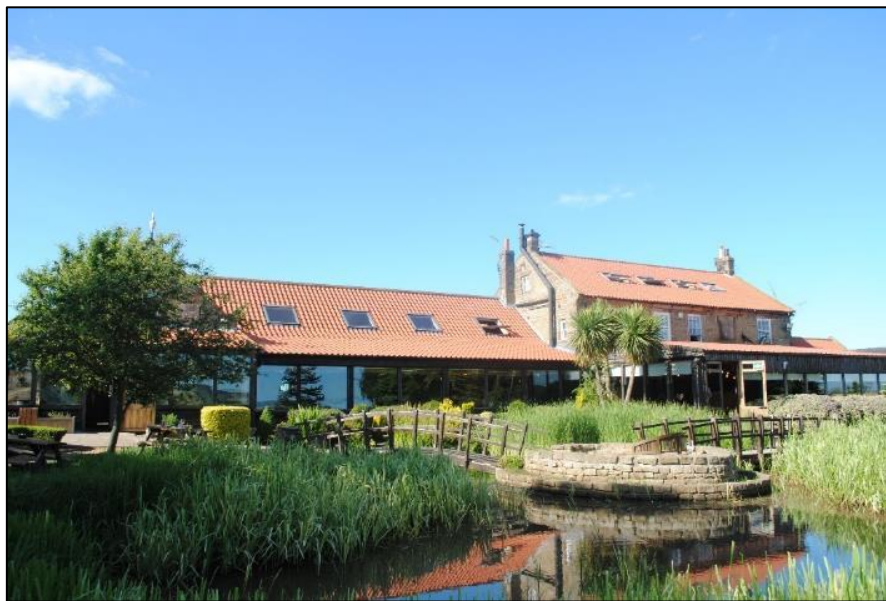
Photo 1. Overview of the buildings from the southwest
