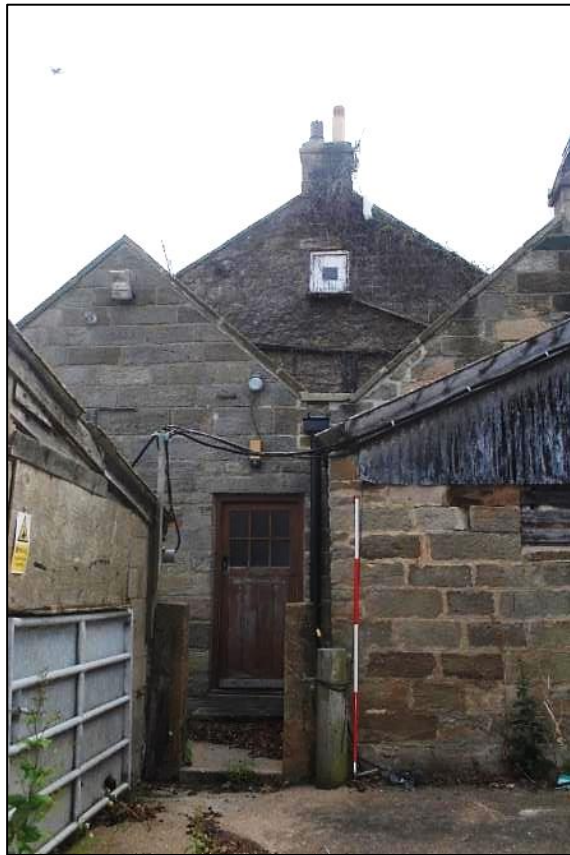
Photo 69. East gable of the Cottage [AB 3]; view west
