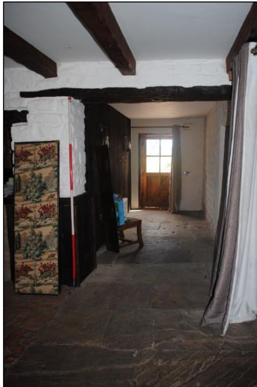
Photo 74. Cottage [AB 3]; south wall; view south
