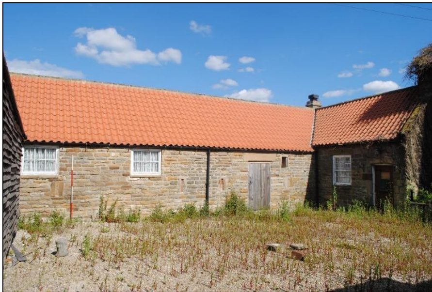
Photo 22. AB 2 west wall; view E/SE from the farmyard
