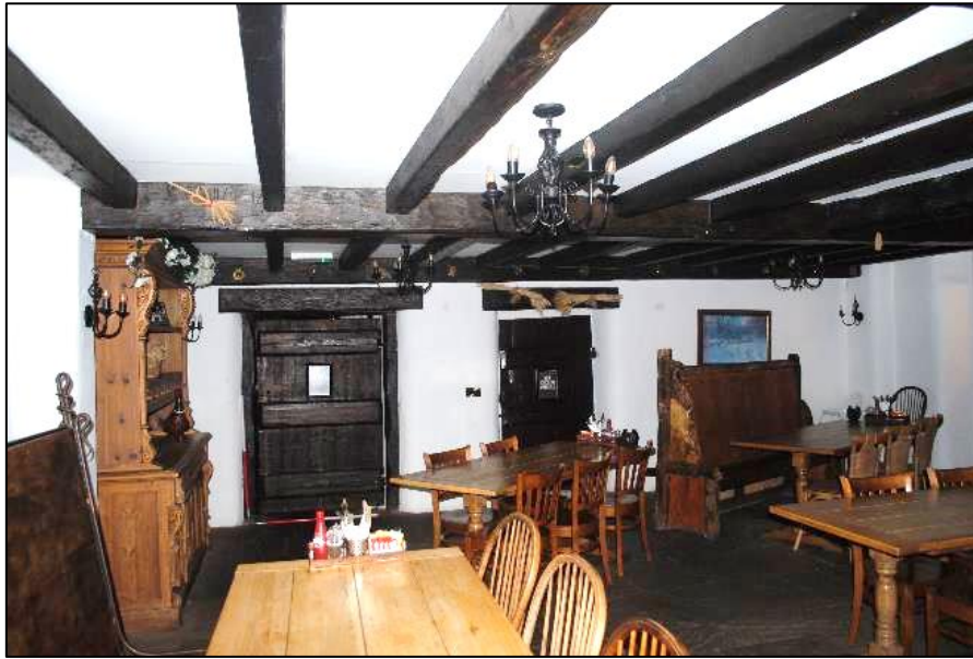
Photo 5. G1 east wall with doors leading to the Cottage [AB 3] and a 20 th century extension
