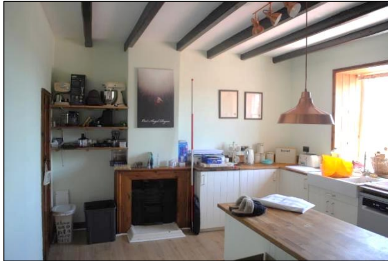
Photo 18. East wall of the kitchen (F2)
