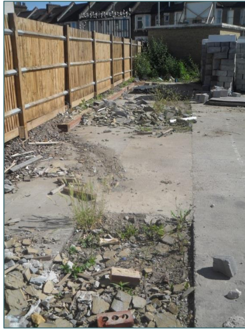
Photo 3: View to the north-east from the proposed development site
