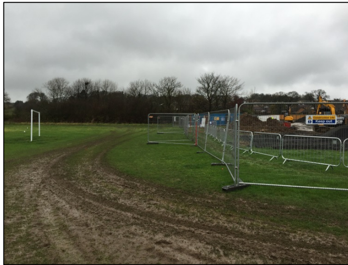
Plate 1: Construction Works along Western Boundary of Site
