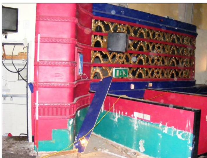
Photo 2: Art Deco moulded plaster proscenium edge and decorative ventilation grill in the auditorium (Scale 2m)
