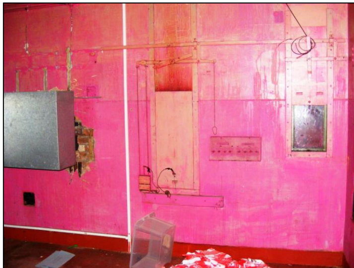
Photo 14: Projection apertures with associated shutter mechanisms. A switch board is visible on the wall between the apertures
