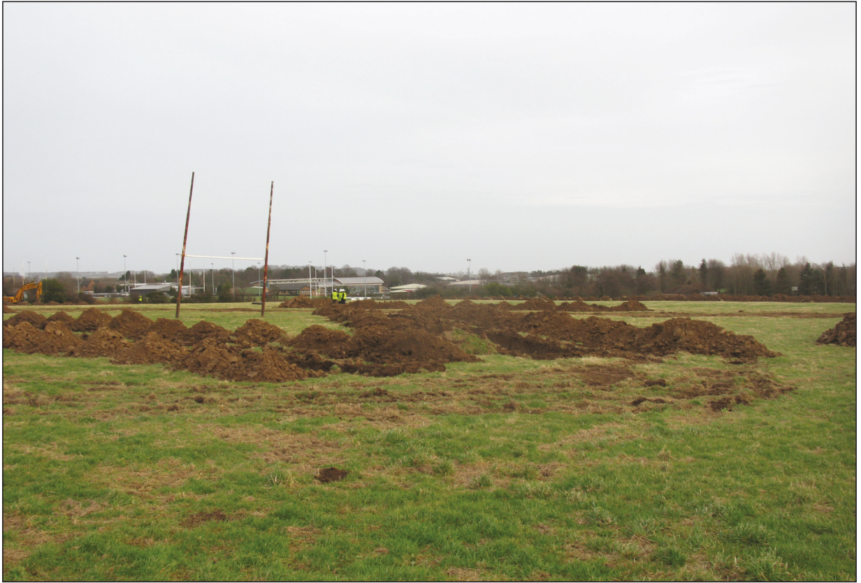
Plate 1 - Working shot of trenches under excavation
