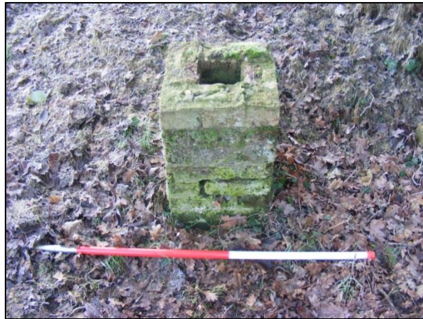
Photo 1: Remains of brick stack (AB 6), viewed from the northeast
