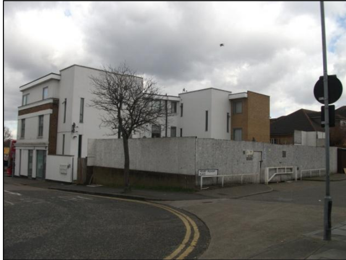
Photo 5: The Proposed Development Site viewed from the south - west
